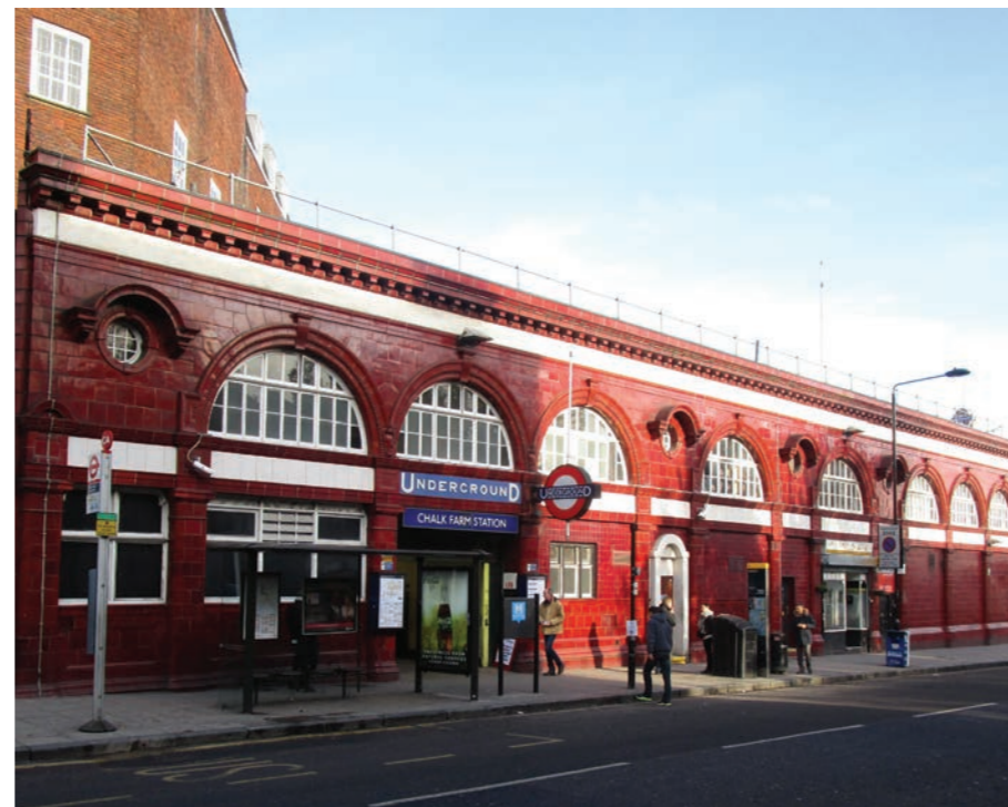
Fig. 7.13: Chalk Farm Station from Adelaide Road, looking south-east.
