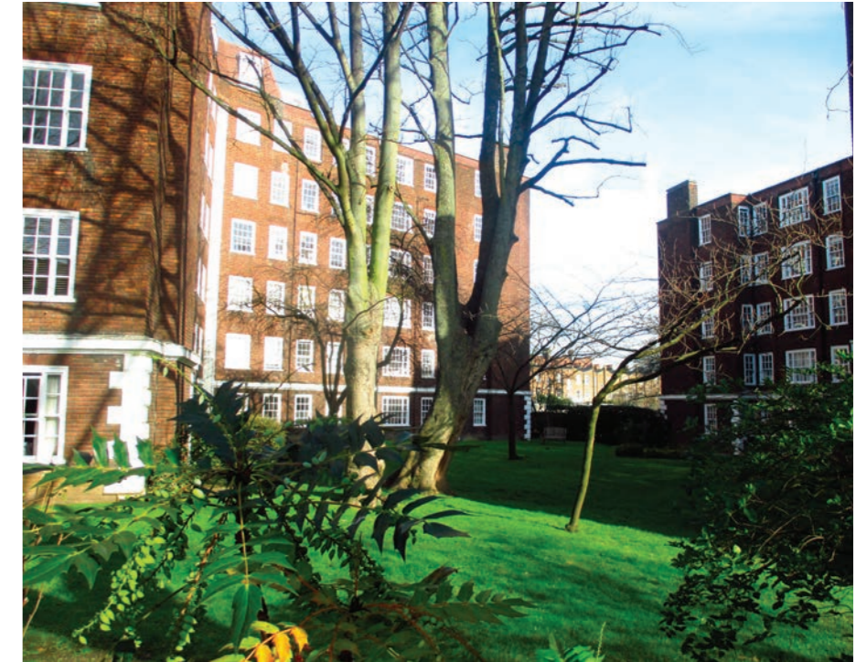
Fig. 4.5: View of Eaton College Road Estates and gardens.
