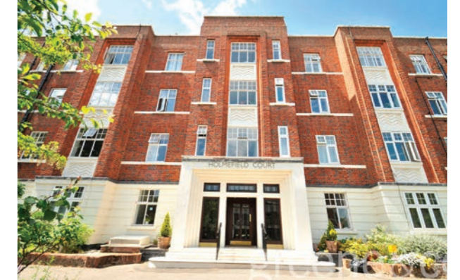
Fig. 3.28: Holmefield Court, Belsize Park
