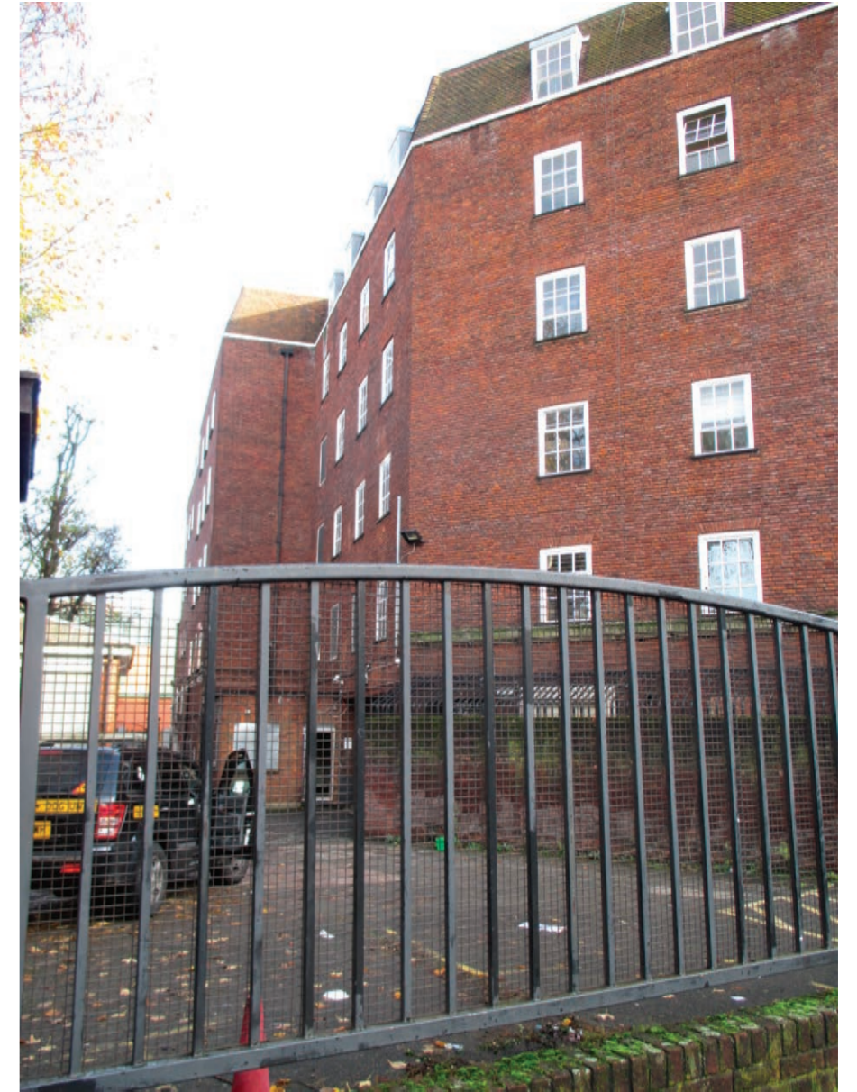
Fig. 4.3: The fenced in area of the site building.
