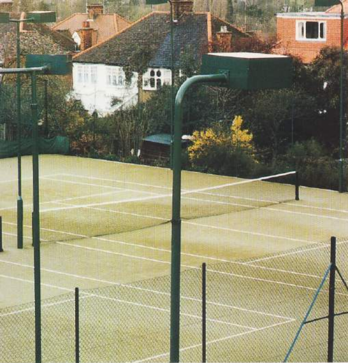
The photographs below were taken from the same position during daytime and evening and shows the minimal glare and light spillage achieved.
