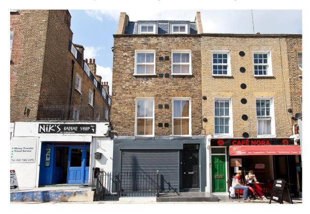
7. The basement is lit by a light well that extends across the whole front of the building. It is accessed externally from stairs in the well - there is no internal access. Two vaults extend out from the light well beneath the road for about 2.6m. The eastern one has an arched entrance.
