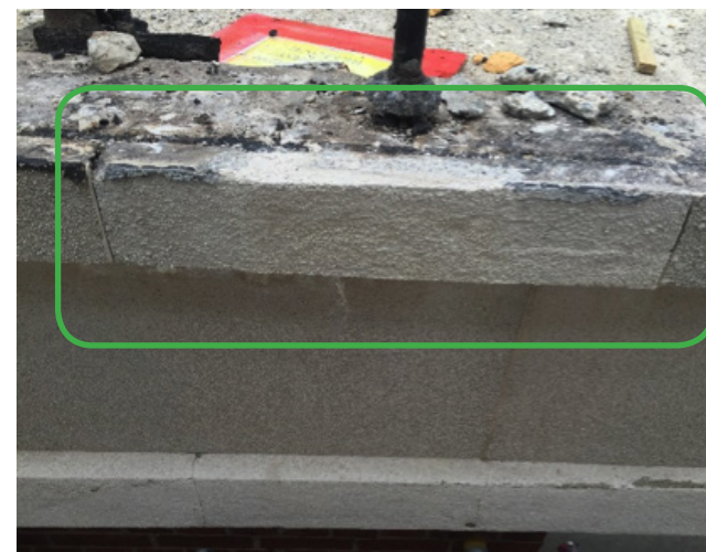
Concrete cill repair after
