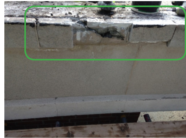
Concrete cill repair before
