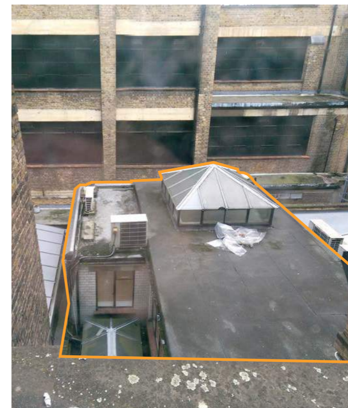
Rear yard in-fill as seen from above
