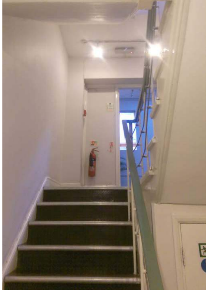
View from stairwell - access to extension at First Floor
