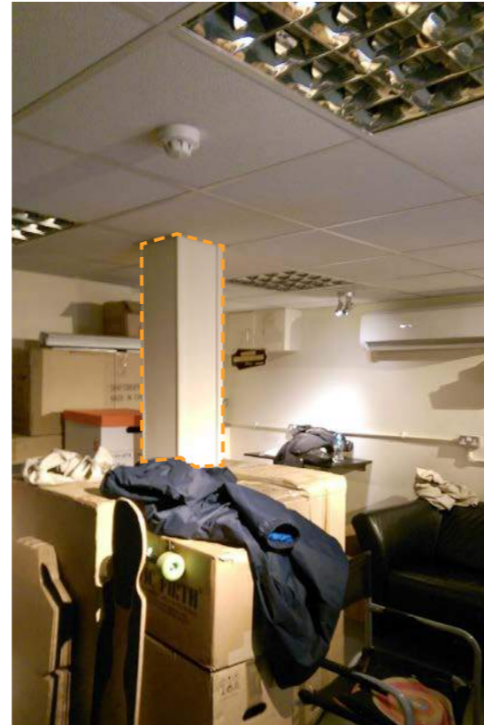
Existing column at Basement level
