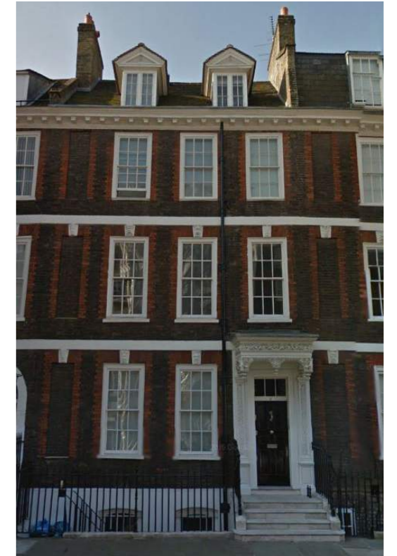
House on Queen Anne's Gate SW1, built in 1700-04 showing typical timber eaves detail with clay roofing tiles of the period
