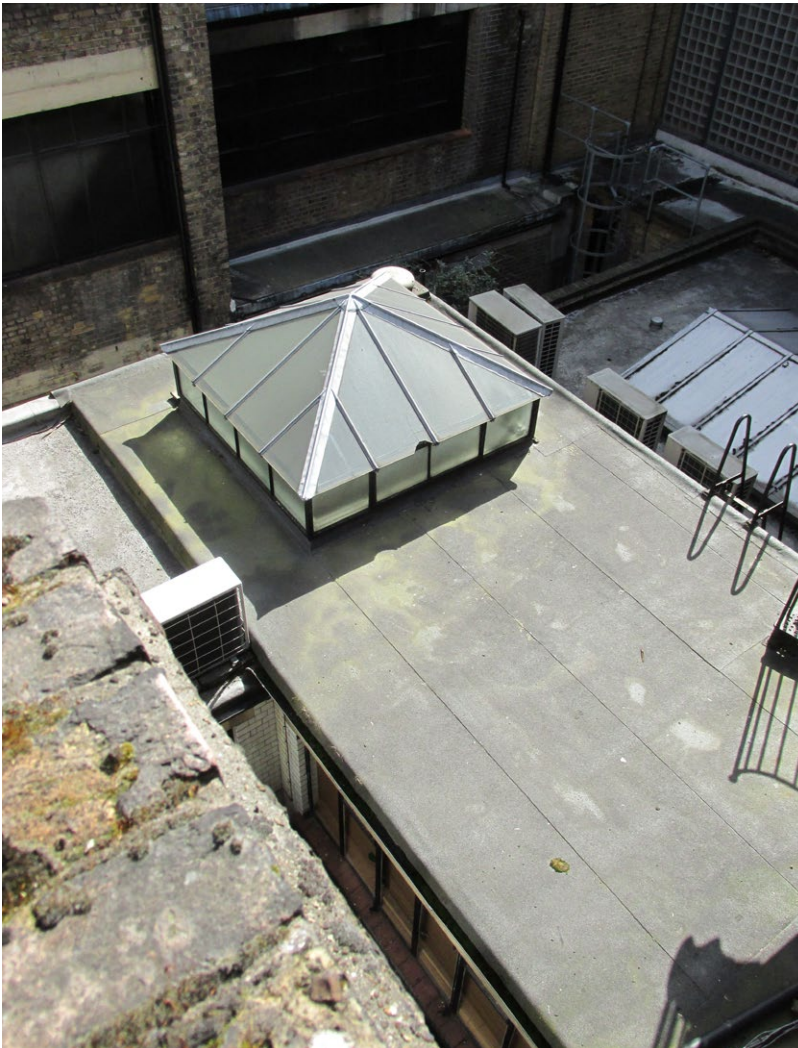
Rear of No. 10 Denmark Street
