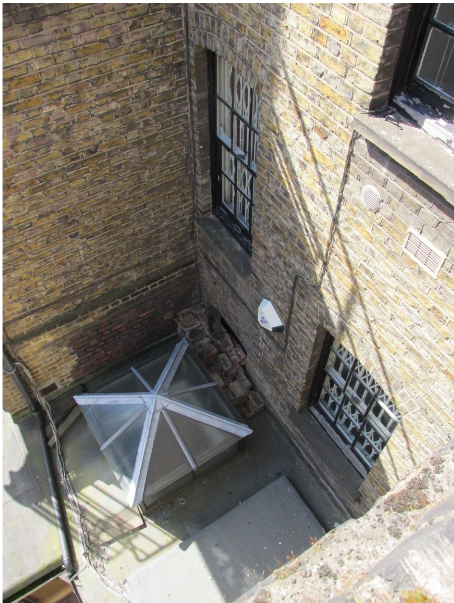
Rear of No. 10, mostly rebuilt in stock brick
