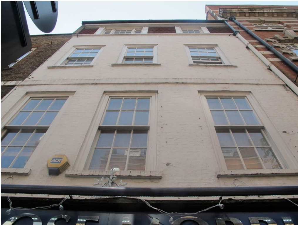
No. 10 Denmark Street frontage
