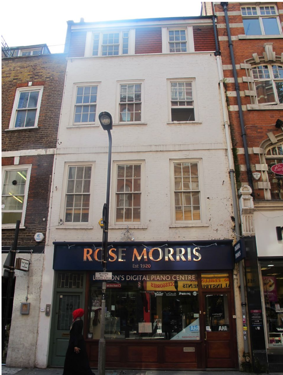
No. 10 Denmark Street, showing twentieth-century shopfront, roof extension and overpainting
