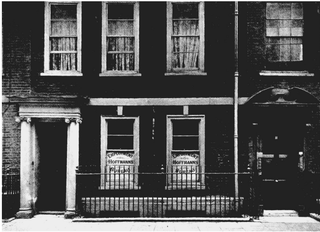
Nos. 10 and 11 Denmark Street, c. 1900. This shows the ground floor of No. 10 before its reconstruction to create a shopfront (Survey of London)
