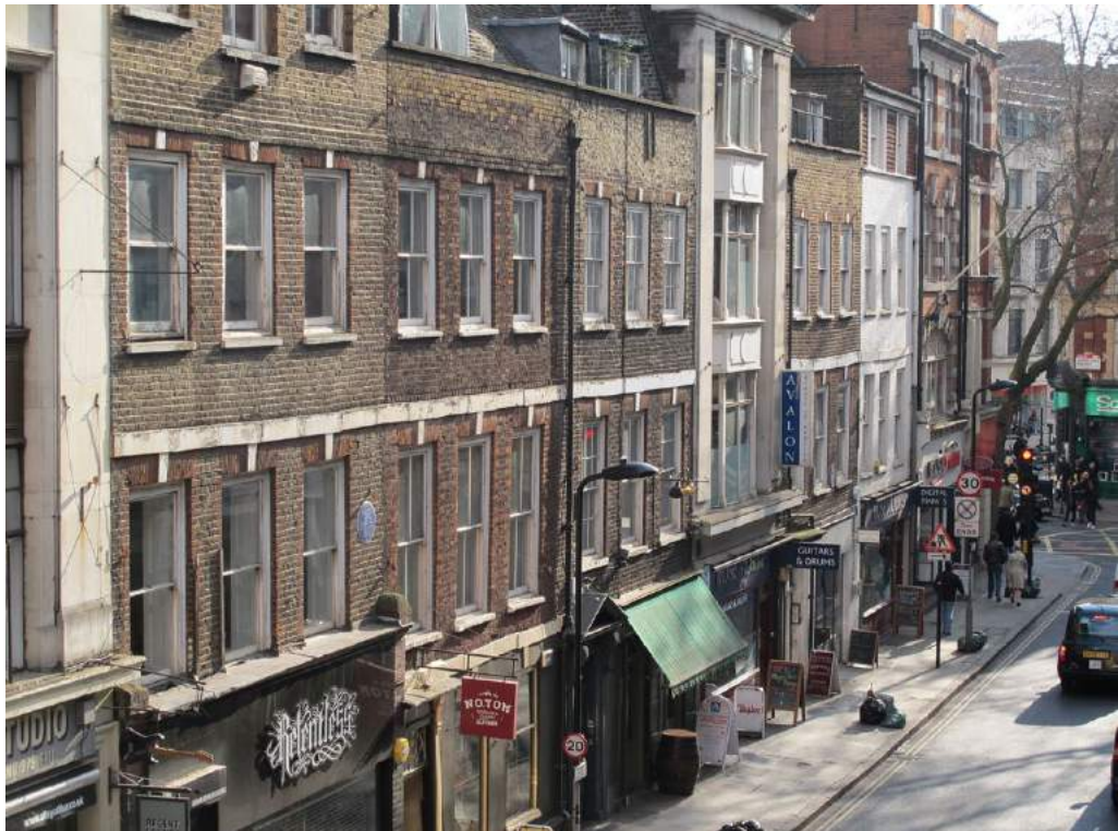
South side of Denmark Street showing Nos. 5, 6, 7, 8, 9 and 10 (painted white). The windows and parapets are not original
