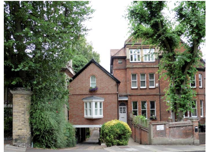
Figure 30. Extant consent for new boundary treatment narrowing vehicular entrance with brick piers and wall App. ref. 2014/331 I/P (38 Netherhall Gardens).
