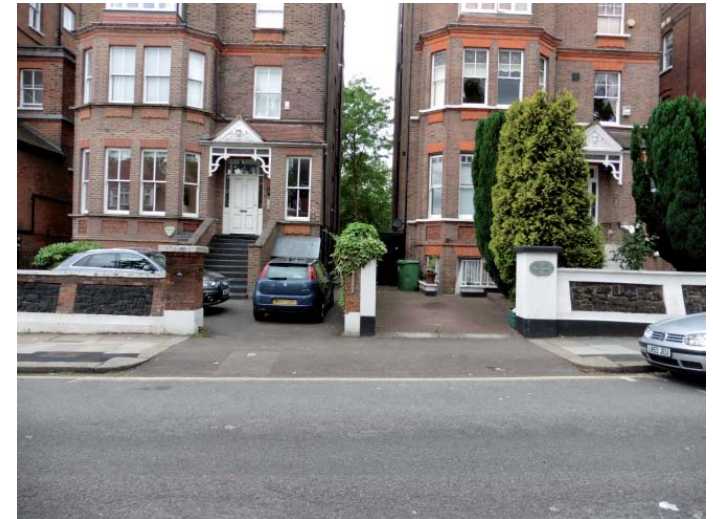
Figure 78. Wide shared crossover with narrow vehicular entrances with tall gate piers and walls. (35 and 37 Maresfield Gardens).
