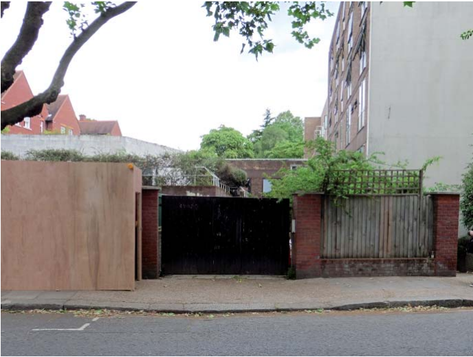
Figure 13. Rear (possibly service) entrance to school with tall brick piers and walls to either side (16 Netherhall Gardens corner in Nutley Terrace).
