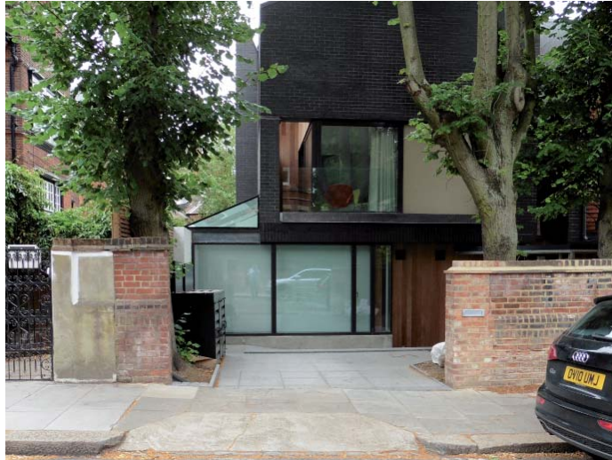
Figure 44. Recently approved redevelopment with high front and side boundary walls and crossover misaligned with driveway (48c Netherhall Gardens App. ref. 2011/1177/P and 2012/4138/P).
