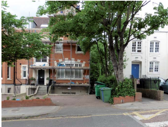
Figure 5. Widened crossover and widened vehicular double entrance. (3 Netherhall Gardens).
