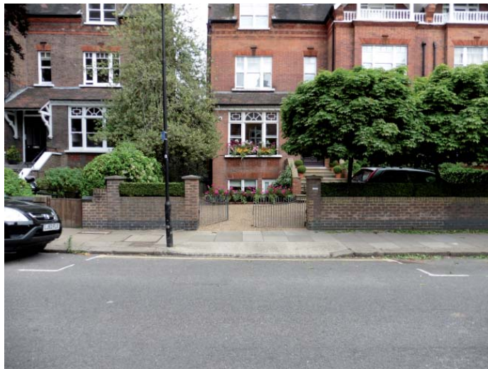
Figure 89. Driveway with brick piers, wall and hedge on either side Previous consent for driveway in alternative position (App. ref. 6/9/B) (10 Maresfield Gardens).
