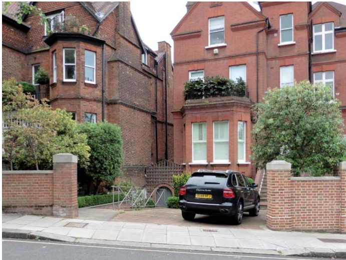
Figure 28. Two sets of tall gate piers and walls frame four off-street parking spaces. 36 Netherhall Gardens. Application Ref. PW9902418.
