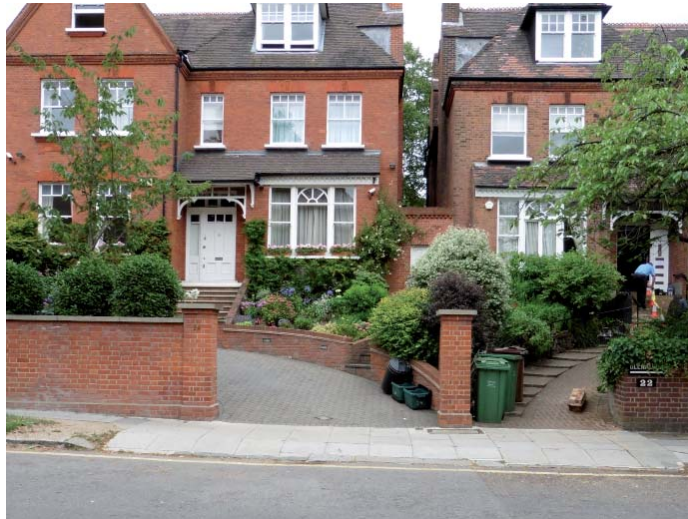
Figure 17. Altered vehicular entrance with high brick piers and walls to either side. Wide crossover. Street tree further obscures sight lines. (24 Netherhall Gardens).
