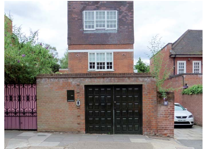
Figure 39. Garage at back of pavement. (48b Netherhall Gardens).
