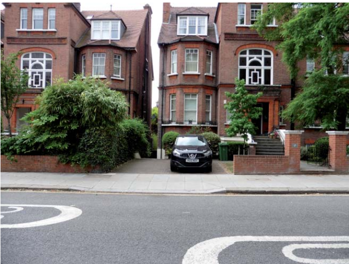
Figure 88. Second of two vehicular access (two of five spaces). Note crossover narrower than driveway width and tall wall/piers to left hand side. App ref. 9100346 (17 Maresfield Gardens).
