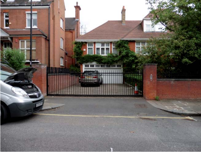
Figure 79. Two car forecourt parking space with driveway width wider than crossover and tall brick piers and walls to either side. App. ref. 2003/2851/C (22 Maresfield Gardens).
