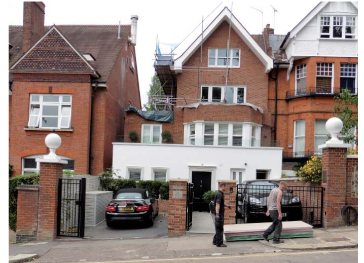
Figure 60. Application property (45 Maresfield Gardens).
