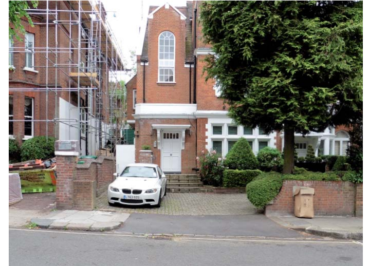
Figure 21. Altered vehicular entrance with wide opening that is wider than crossover in front (28 Netherhall Gardens).
