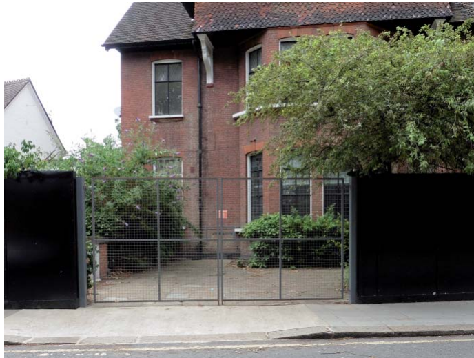
Figure 11. Widened vehicular entrance off-set from crossover/dropped kerb position (Otto Schiff House Netherhall Gardens / corner of Nutley Terrace).
