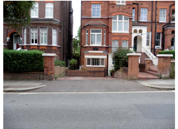
Figure 84. Double width forecourt parking space with wide crossover and tall brick piers to either side. App ref. 33897 (27 Maresfield Gardens).
