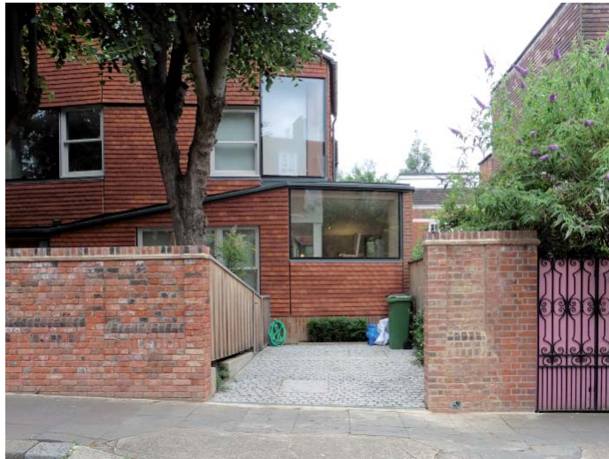
Figure 41. Recently approved redevelopment for development of two new houses with narrow entrance, high walls to either side, and crossover misaligned with driveway. App. Ref. 2010/1946P 48b Netherhall Gardens.
