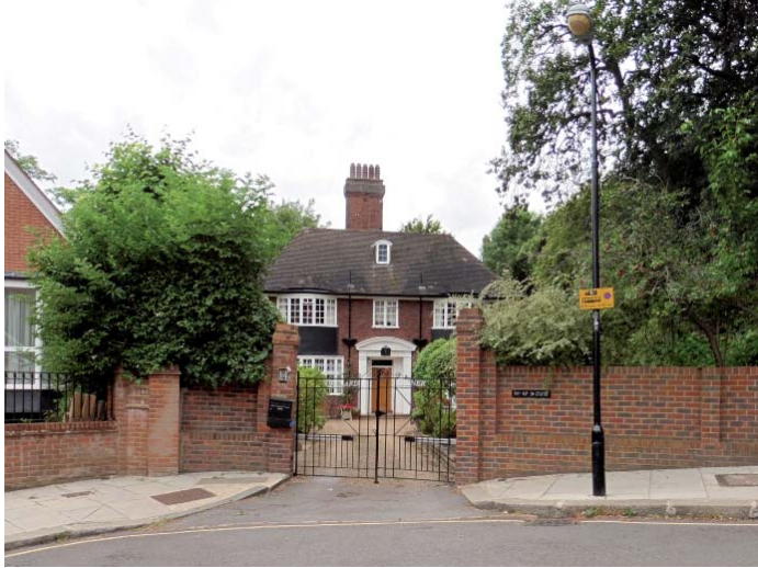
Figure 25. Narrow entrance with high piers and walls to either side. Consent granted for substantial redevelopment including basement car park without alterations to driveway. (Orchard Corner, Netherhall Gardens) Application Ref. 2006/4031/C and PWX0102124.
