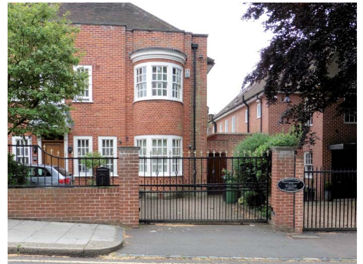
Figure 36. Gateway narrowed and inset gate piers constructed. Note wider crossover in front and spreading in from of adjacent driveway. Single pier separate driveway to the right ( mirroring lefts hand side entrance see next photo) (44 Netherhall Gardens).
