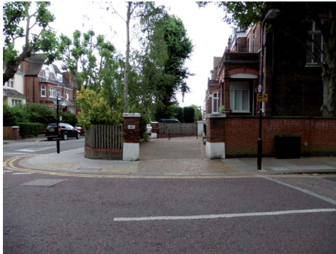
Figure 68. One of two vehicular entrances, this one very close to road junction (41 Maresfield Gardens).
