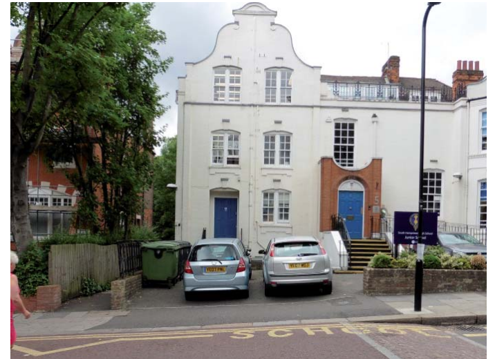
Figure 6. School with widened crossover and widened double entrance at 'School' markings on the highway (5 Netherhall Gardens).
