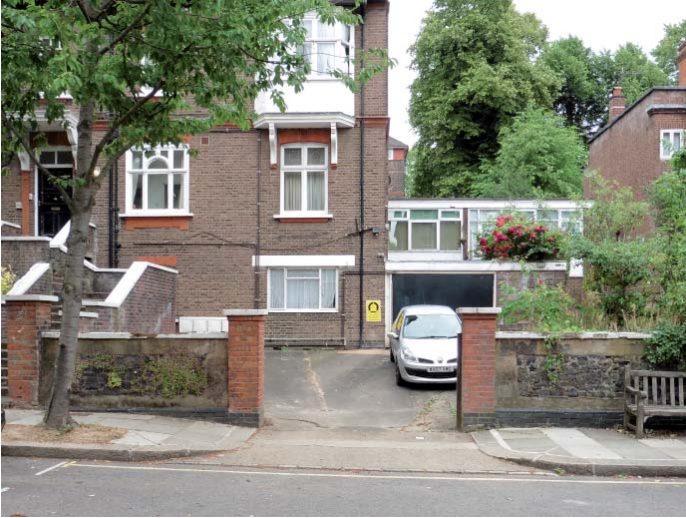
Figure 19. Unaltered vehicular entrance with high walls and piers serving multiple surface parking spaces and a garage (Netherhall Gardens).
