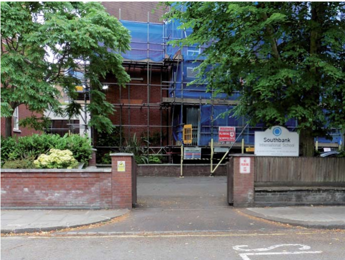
Figure 16. School entrance also serving as pedestrian entrance (16 Netherhall Gardens).
