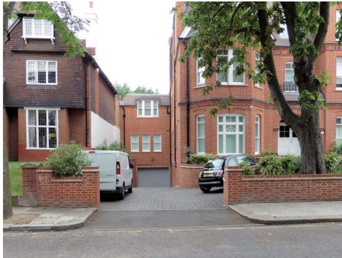
Figure 14. Redevelopment with two vehicular entrances retained but serving separate parking areas. (Samara Mansions 11 Netherhall Gardens).
