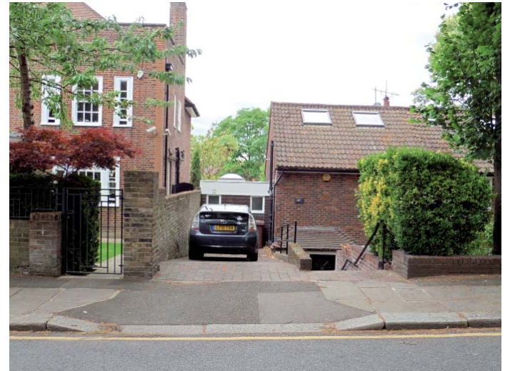
Figure 51. Narrow driveway with tall brick piers to left hand side (55 Maresfield Gardens).
