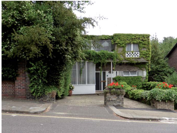
Figure 62. One of two driveways (48 Maresfield Gardens).
