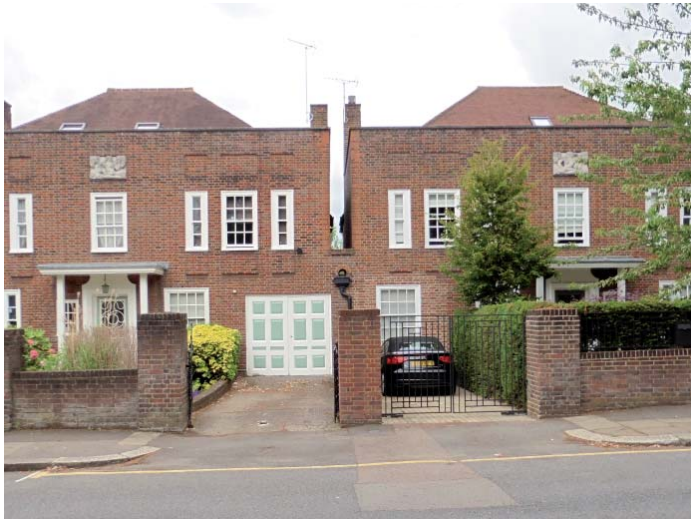
Figure 52. Narrow driveways with tall brick piers on either side and combined crossover, Combined crossover. (51 & 53 Maresfield Gardens).
