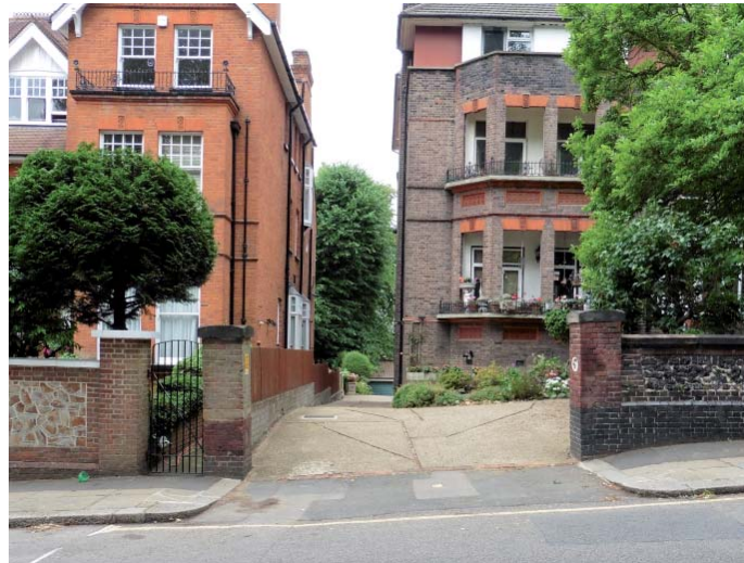
Figure 59. Wide entrance with tall piers and walls accessing front and rear parking areas and garages. Note 47 has a further vehicular entrance to the right hand side (47 Maresfield Gardens).
