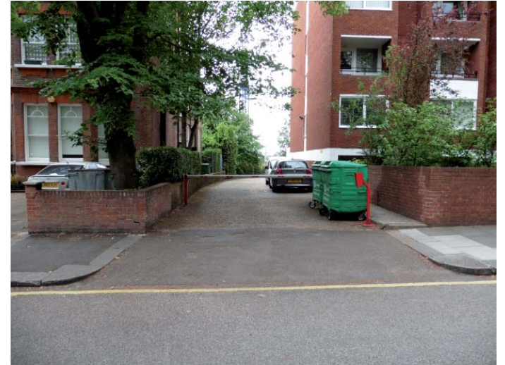
Figure 93. Automatic barrier positioned close to back of pavement resulting in entering vehicles parking across the footpath. Also note position of paladin bins to right hand side (11-13 Maresfield Gardens).
