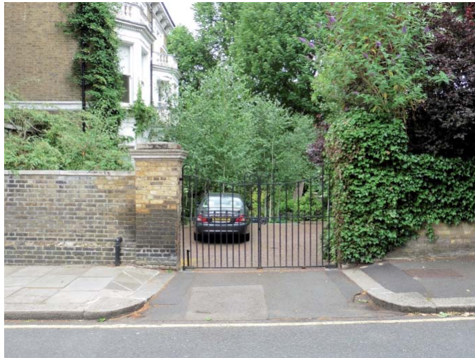
Figure 47. Narrow driveway with tall brick piers and wall (40 Netherhall Gardens).
