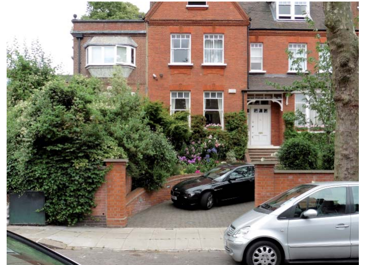
Figure 18. Altered vehicular entrance with high brick piers and walls to either side. Wide crossover. Street tree further obscures sight lines. (24 Netherhall Gardens)
