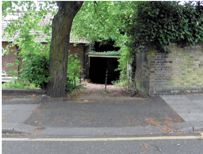
Figure 50. Narrow driveway with tall brick wall to one side and mature tree to the left (59 Maresfield Gardens).
