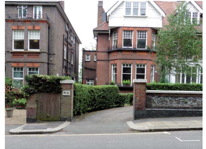
Figure 57. Second entrance to 49 with tall gate piers and walls (49 Maresfield Gardens).
