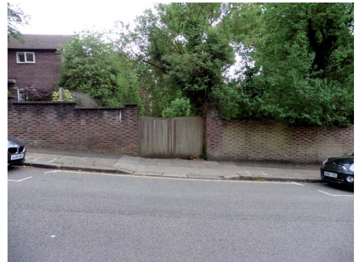
Figure 66. Narrow vehicular access with tall gate piers and walls (46 Maresfield Gardens).
