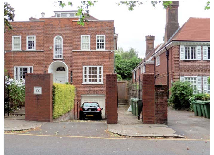
Figure 48. Narrow driveway with tall brick piers and wall (70 Maresfield Gardens)
