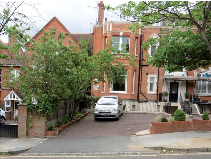
Figure 4. Widened crossover and widened vehicular double entrance. (3 Netherhall Gardens).
