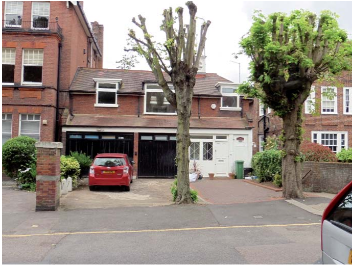
Figure 55. Triple crossover (without front of pavement kerb line) serving up to three properties with tall gate piers and mature trees. (51 Maresfield Gardens).
