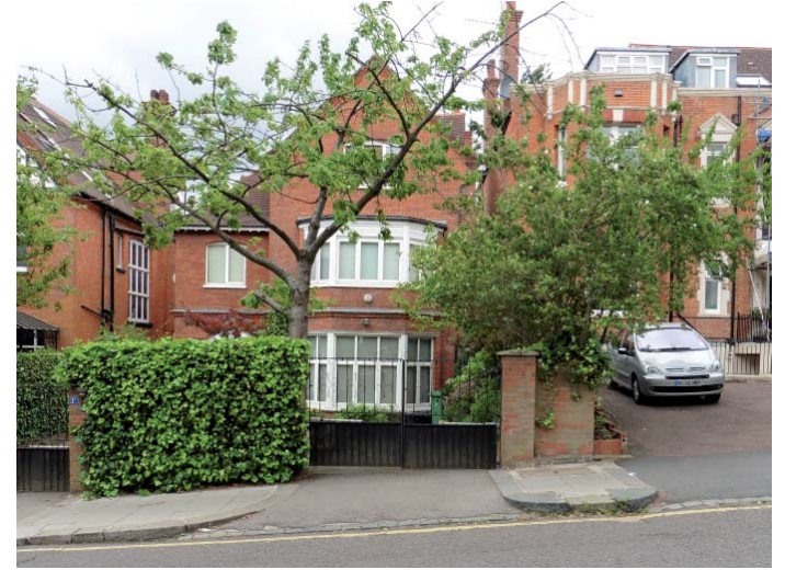
Figure 3. Double vehicular entrance to single property with tall brick piers and boundary wall (1a Netherhall Gardens).
