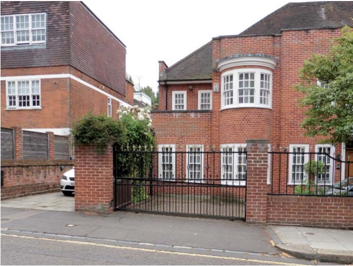
Figure 37. Second of two vehicular entrances with tall piers and in close proximity to adjacent driveway to the left with shared crossover (44 Netherhall Gardens).
