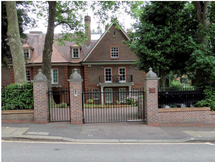
Figure 58. Narrowed gateway with tall brick piers to either side. Note post boxes fixed to railings to right hand side. Note gateway narrowed in relation to crossover (52 Maresfield Gardens).
