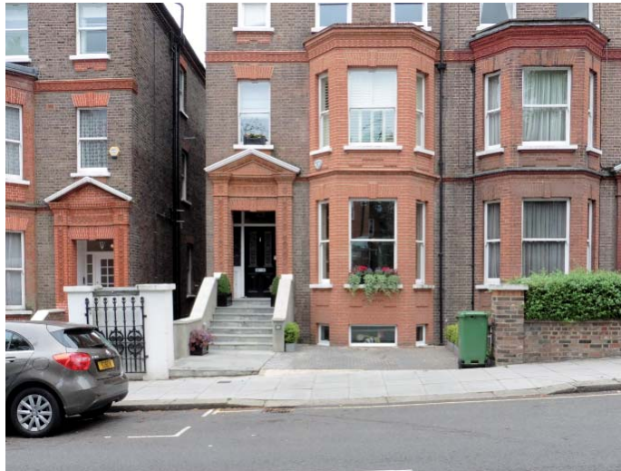
Figure 23. Crossover and hardstanding formed with boundary treatment lost. Parking space is insufficiently deep so that cars may overhang the pavement (29 Netherhall Gardens).
