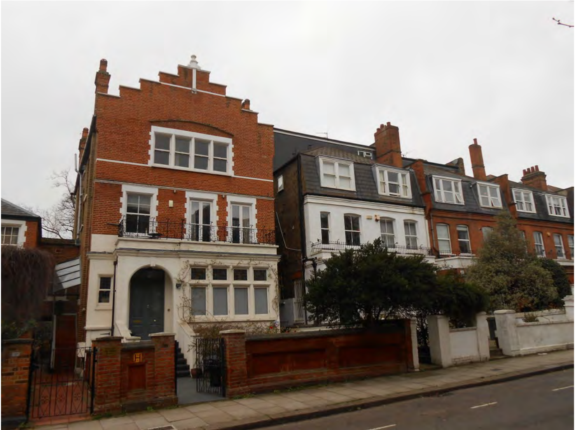
Appendix 2.18: Detached house, South Hampstead Conservation Area
