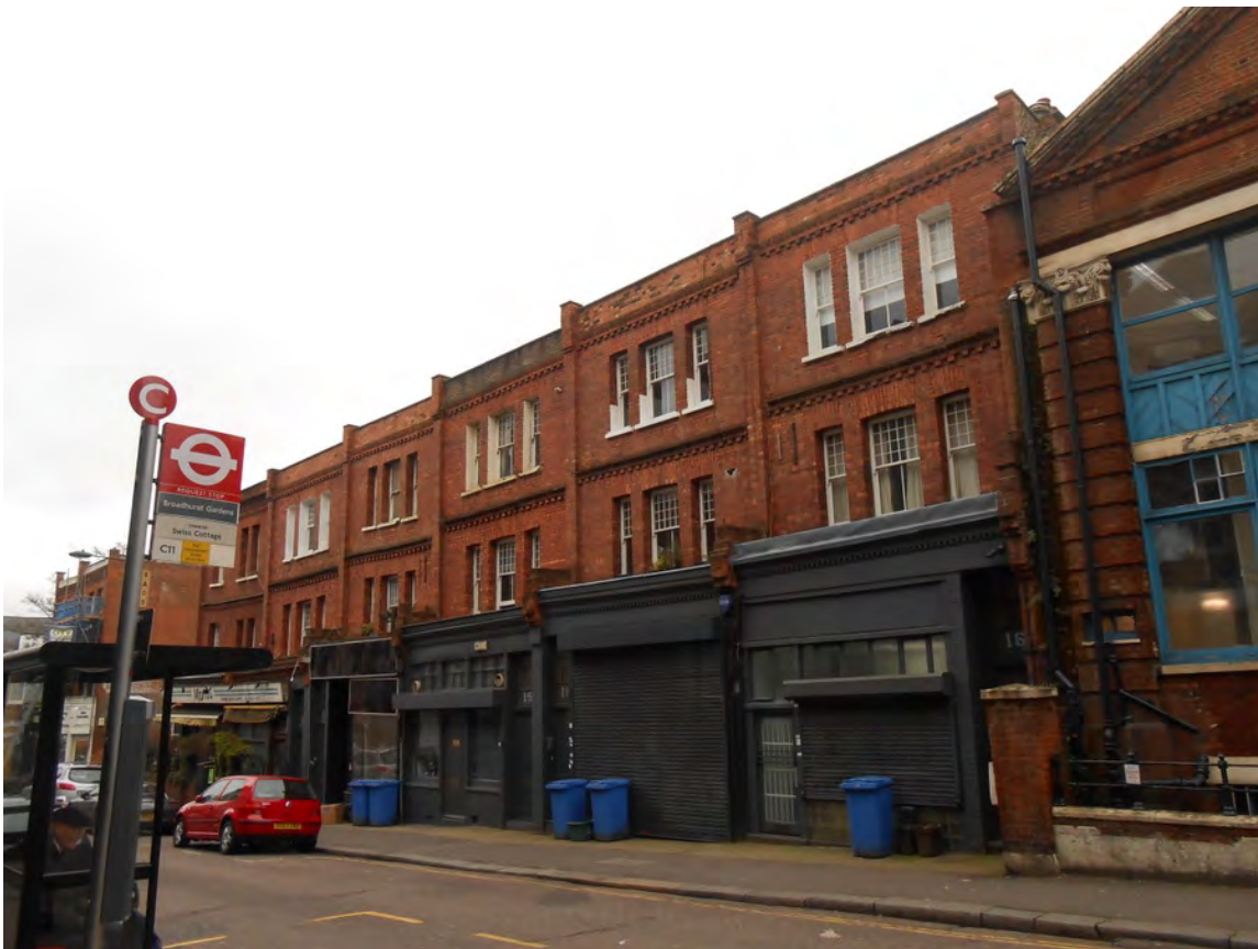
Appendix 2.2: View of Application Site from Broadhurst Gardens looking south-east
