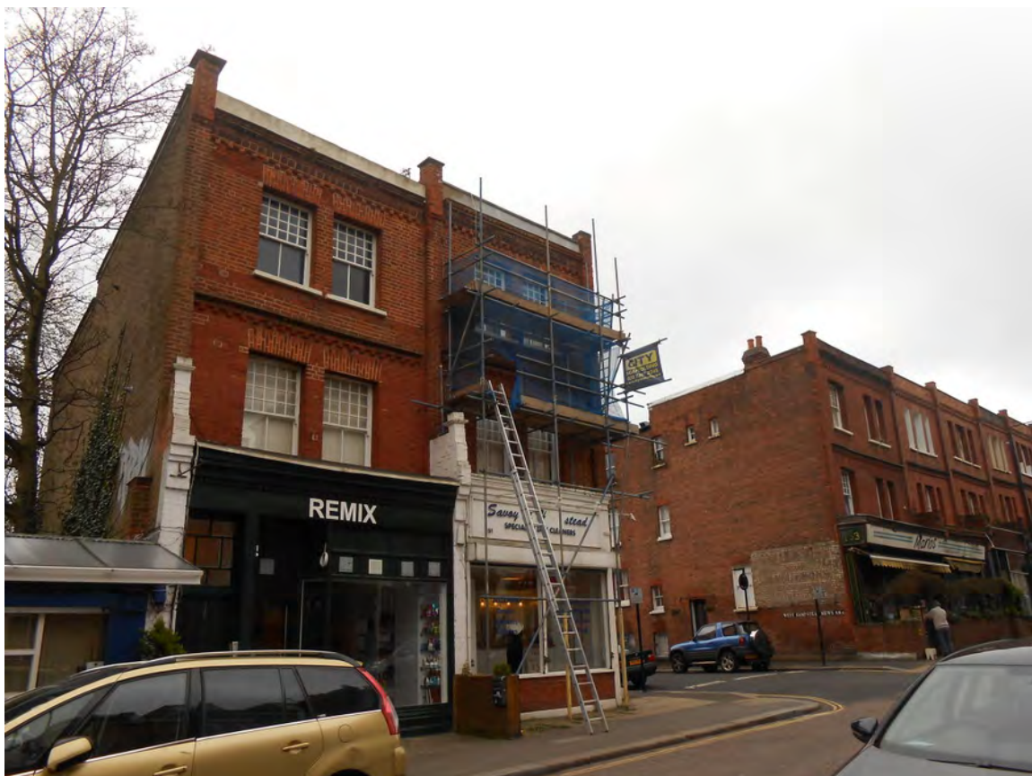
Appendix 2.16: View of properties on eastern side of West Hampstead Mews, looking south-west.
