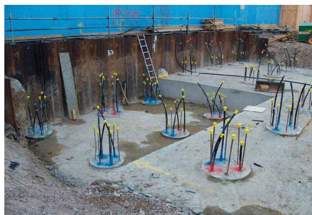
Energy piles within foundations of construction. Source: Geothermal International Italia
