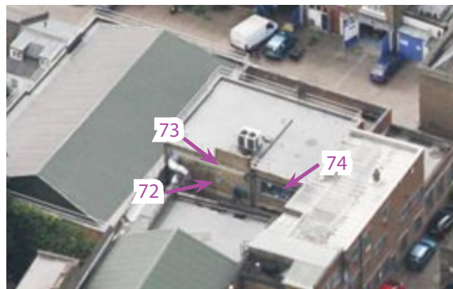
Windows on 165-167 Broadhurst Gardens
