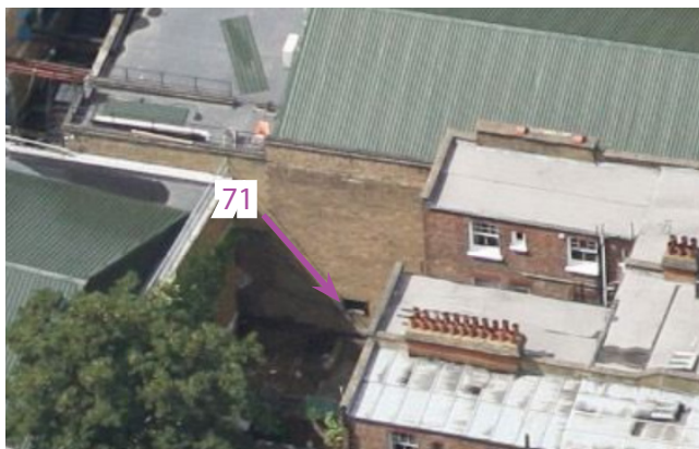
Windows on 165-167 Broadhurst Gardens
