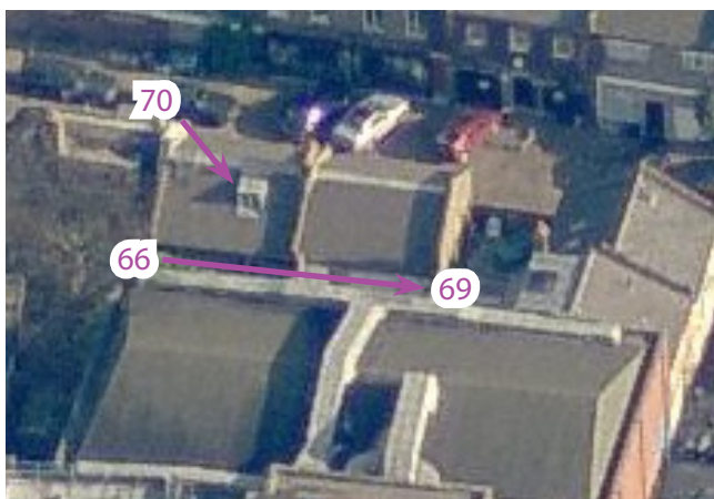
Windows on 22 West Hampstead Mews
