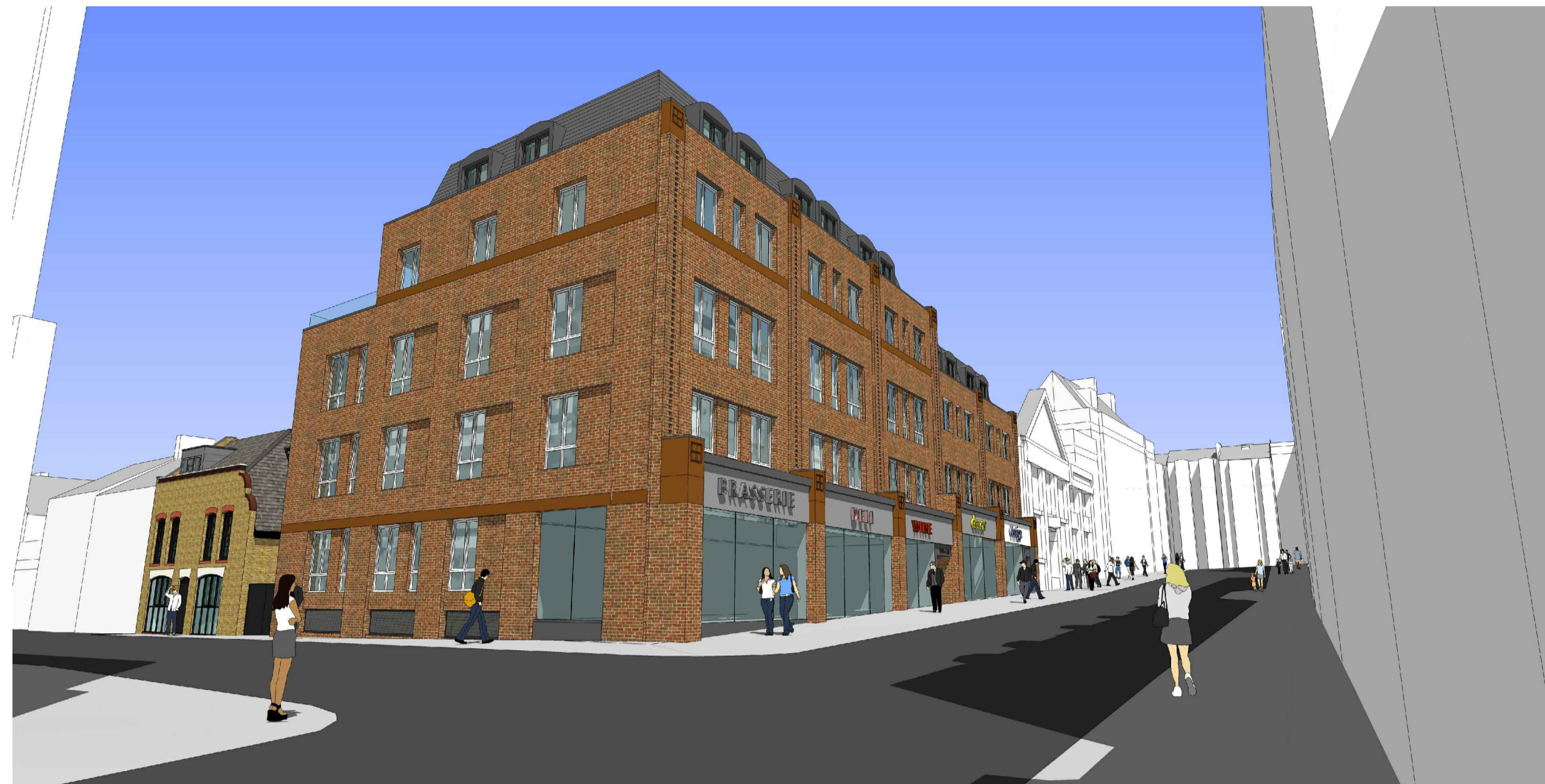
VIEW WEST UP BROADHURST GARDENS
