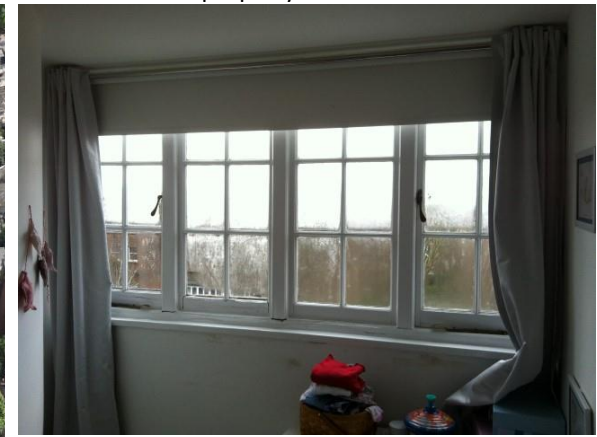
View of the dormer window from inside the room
