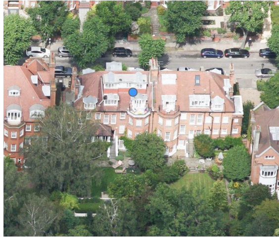
Rear View of the property
