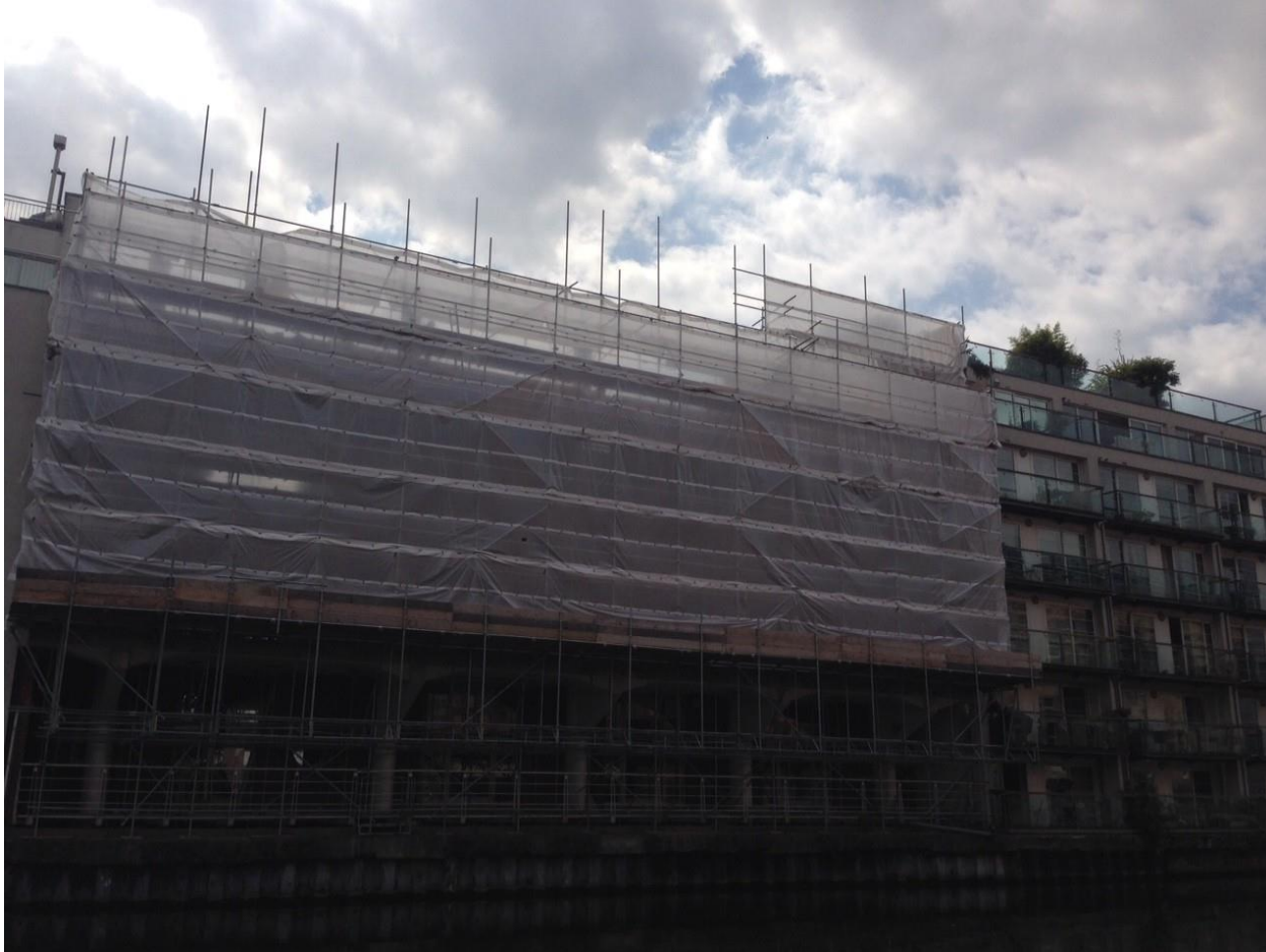
View from Site currently under construction
