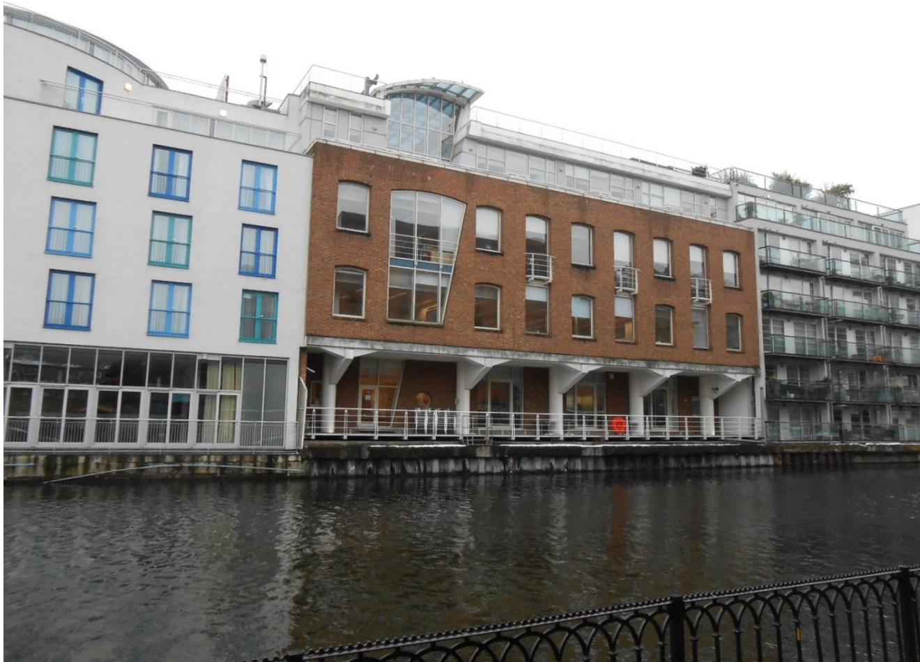
View from Canal towpath
