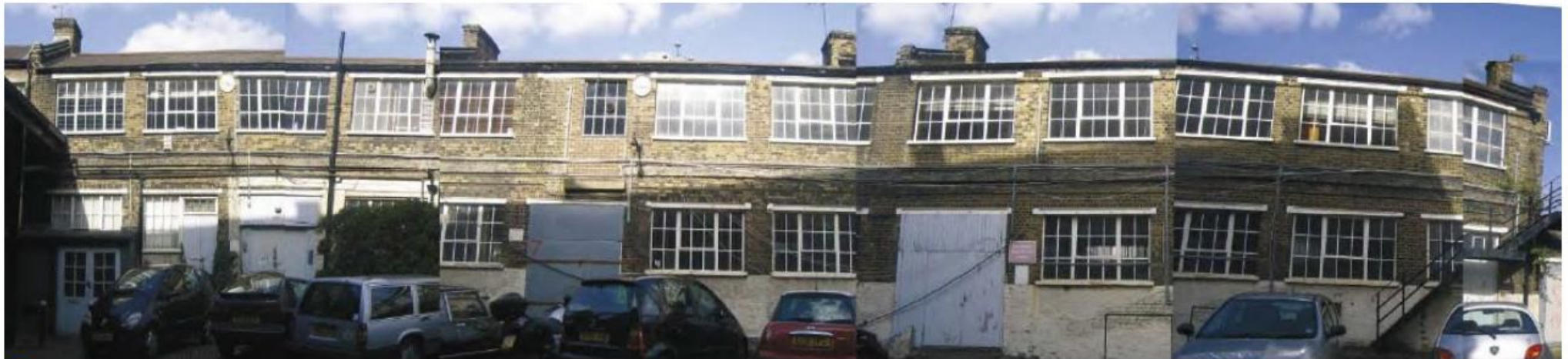
C INDUSTRIAL BUILDING ON THE RAILWAY TRACK BOUNDARY.
