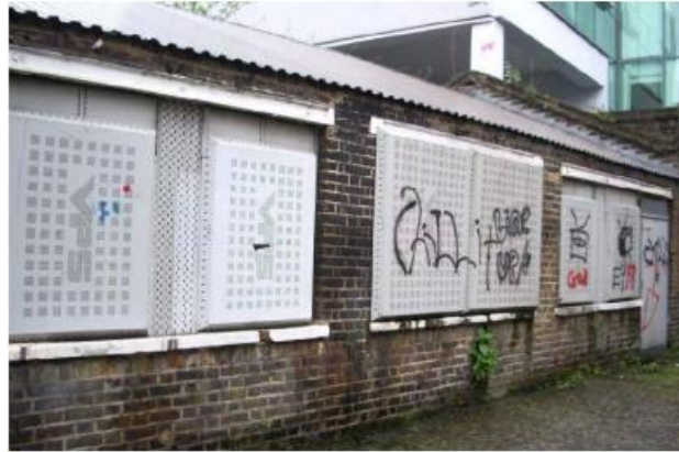
D COURTYARD FACING BUILDING. (DEMOLISHED WITHIN CONSENTED 2012 SCHEME)
