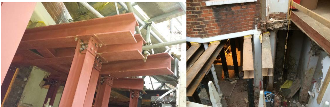
Figure 1 Example of needling to existing wall
