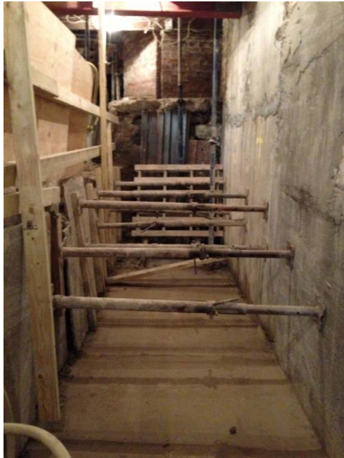
Figure 5 Examples of completed walls and back propping to central soil mass
