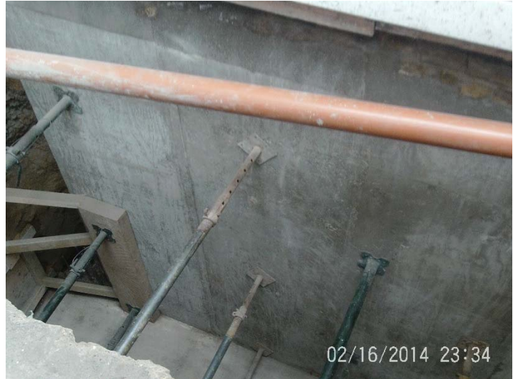
Figure 5 Examples of completed walls and back propping to central soil mass
