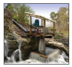
In a residential small scale hydro system the constant flow of water is critical to the success of the project. The energy available from a hydro turbine is proportional to the flow rate of the water and the head height. Since the majority of the cost of a small hydro project stems from up front expenses in construction and equipment purchase, a hydro project can generate large quantities of electricity with very low operating costs and modest maintenance expenditures for 50 years or longer.
