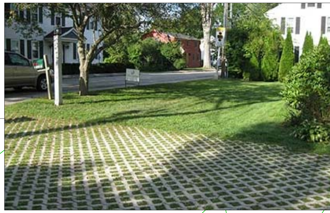
Sample of Permeable Paving
