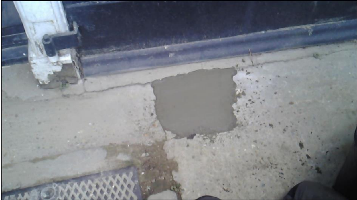
Image 3: Showing the BH upon completion
