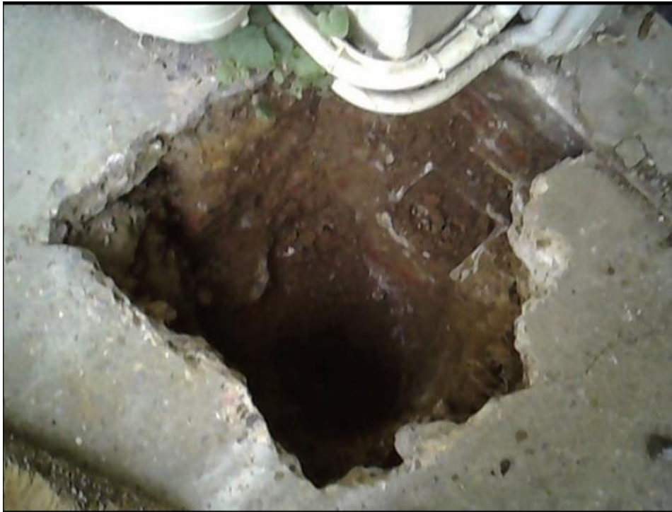
Image 4: showing TP/BH2 open prior to completion
