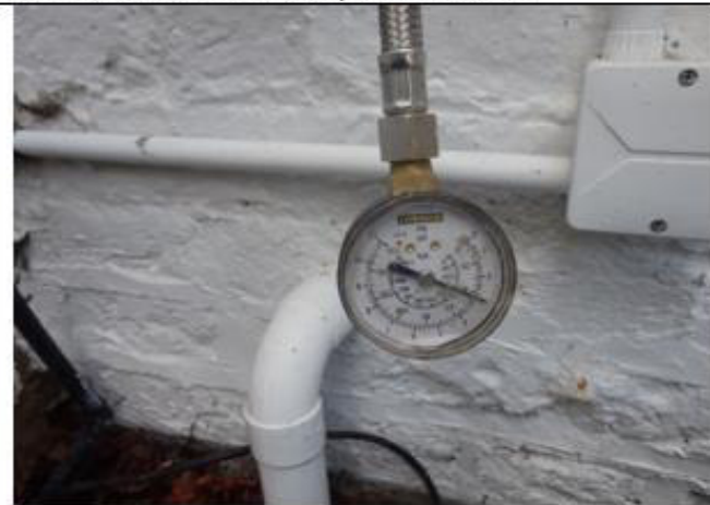
5. Mains water pressure test.
