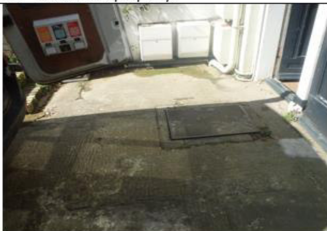
17. Front surface area.
