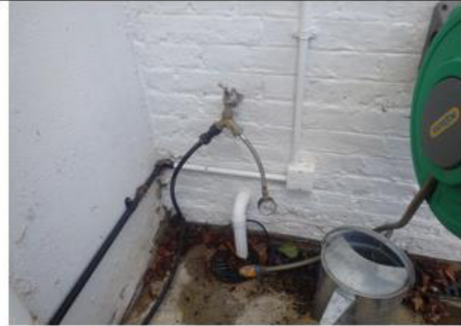
3. FWG1/Mains water pressure test.
