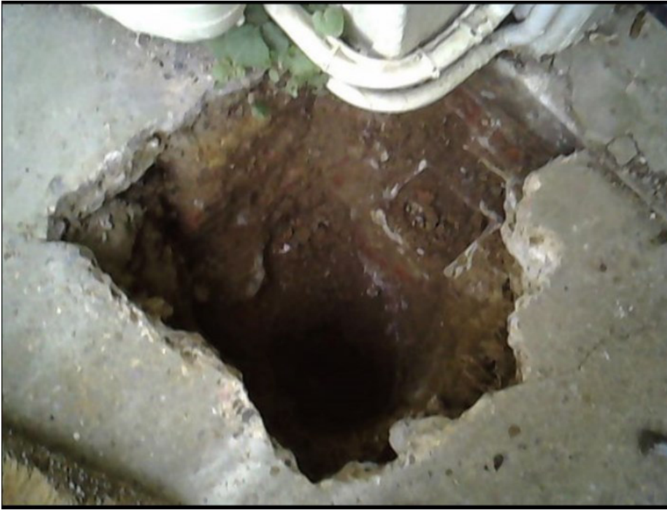
Image 1: showing TP/BH2 open prior to completion
