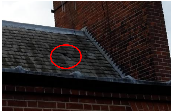
Photograph 4 Missing tile on the western elevation of B2
