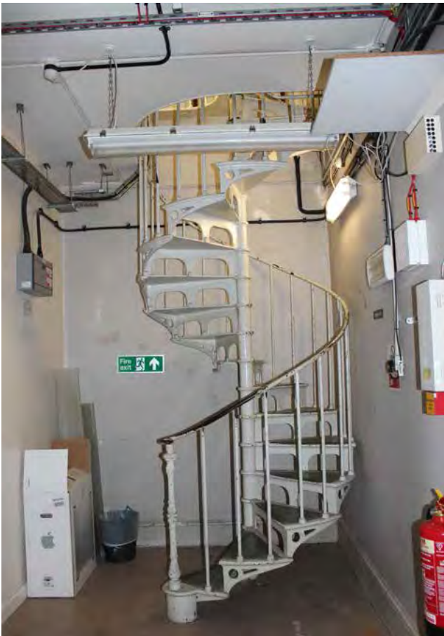
Figure 19: Existing spiral metal stair to be removed, new slab infill where staircase is removed.
