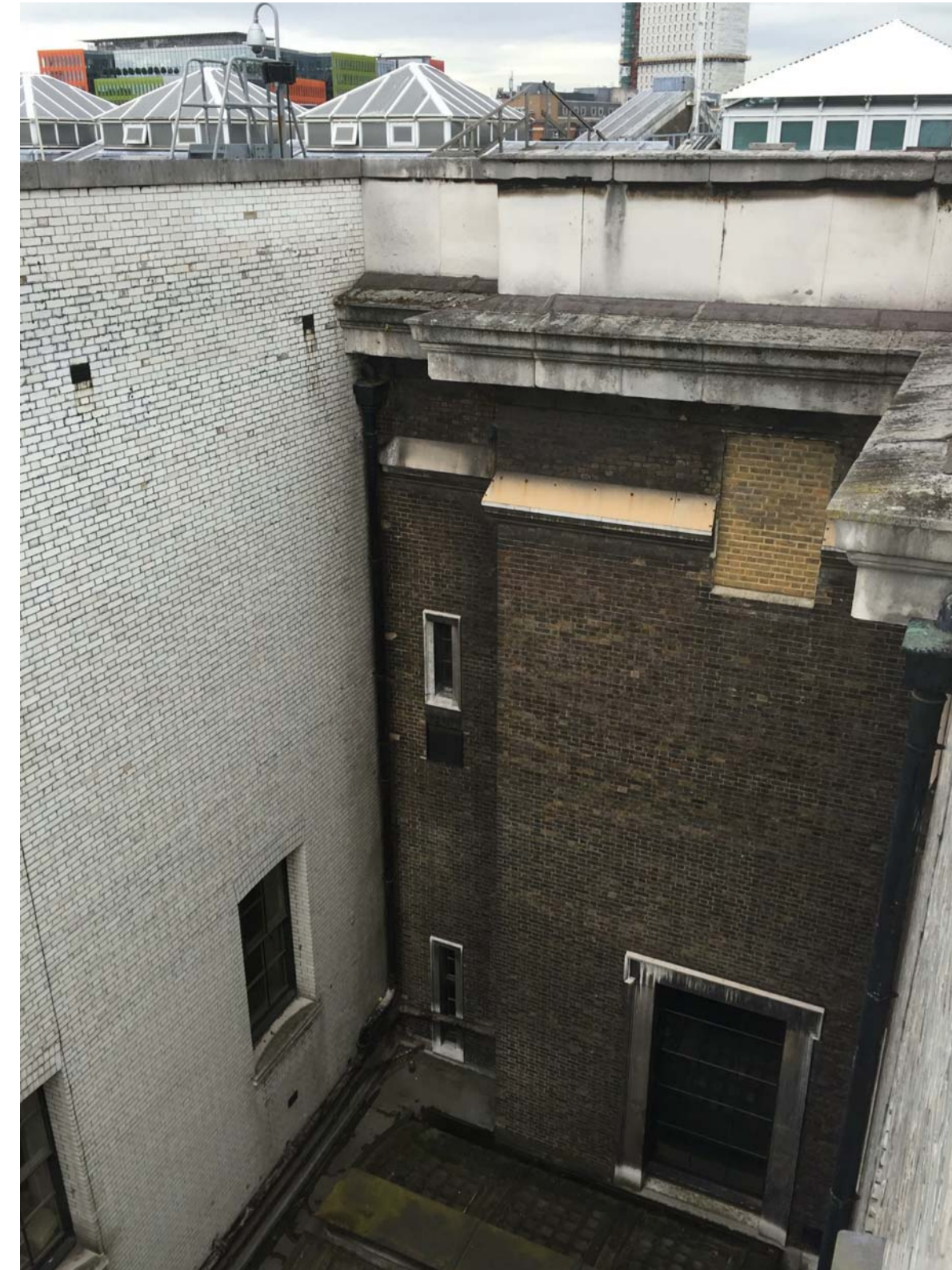
VIEW OF COURTYARD WEST FACADE
