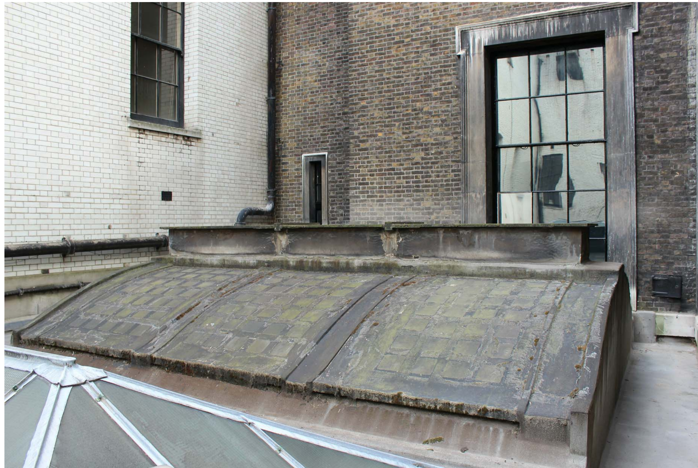
HEAVILY PROPPED CONCRETE VAULT ROOF TO BE DEMOLISHED
