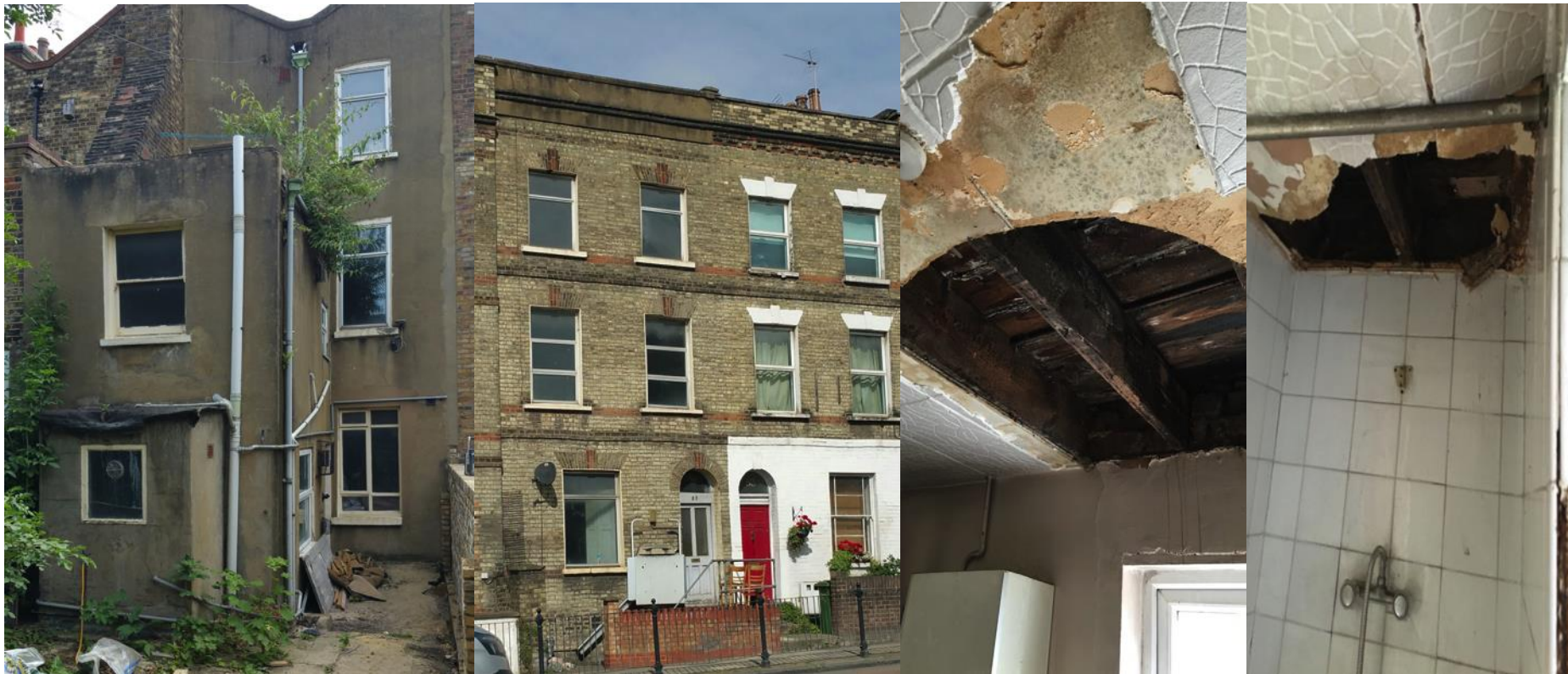
Back extension to existing property
