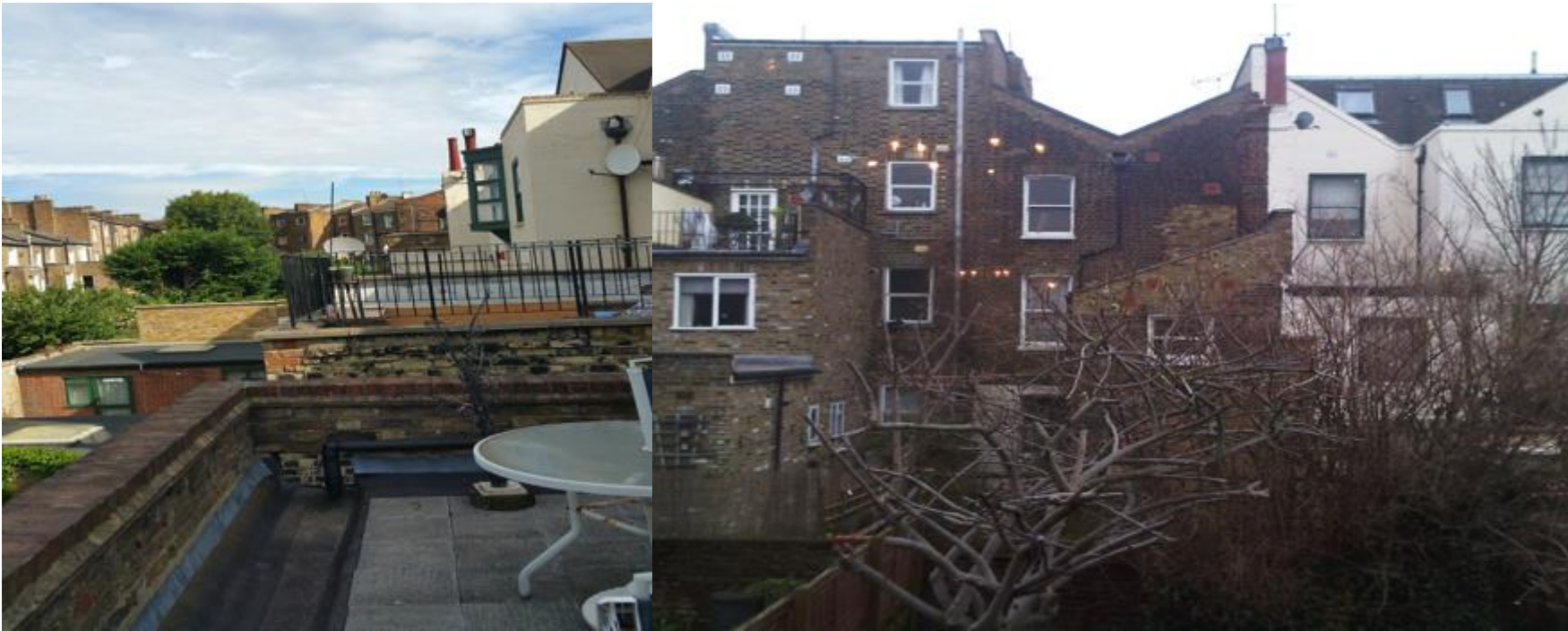
Existing terraces and ground floor extensions 83-93 York Way / Extensions/terraces and mansards of no.89 and 93, prior to no.91 mansard
