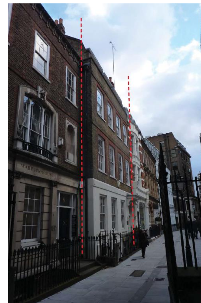
Existing Front Elevation of 7 Warwick Court
