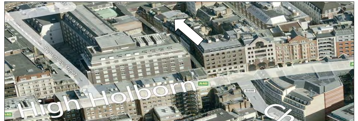
Figure 3: Site Aerial View of 7 Warwick Court
