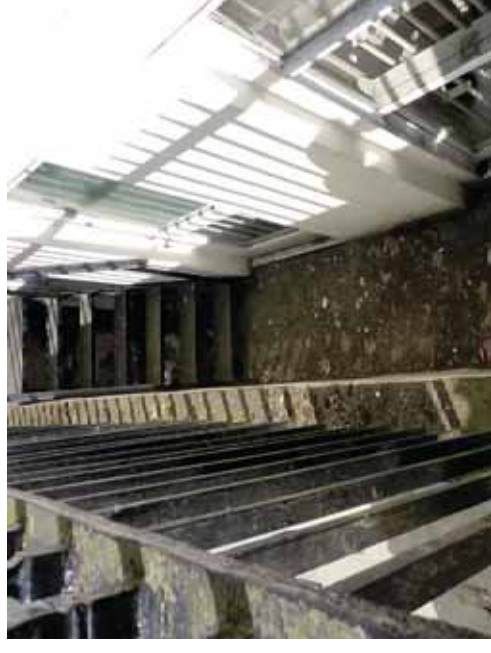
7 Warwick Court Front Lightwell
