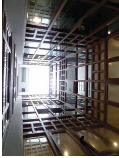
7 Warwick Court Lightwell
