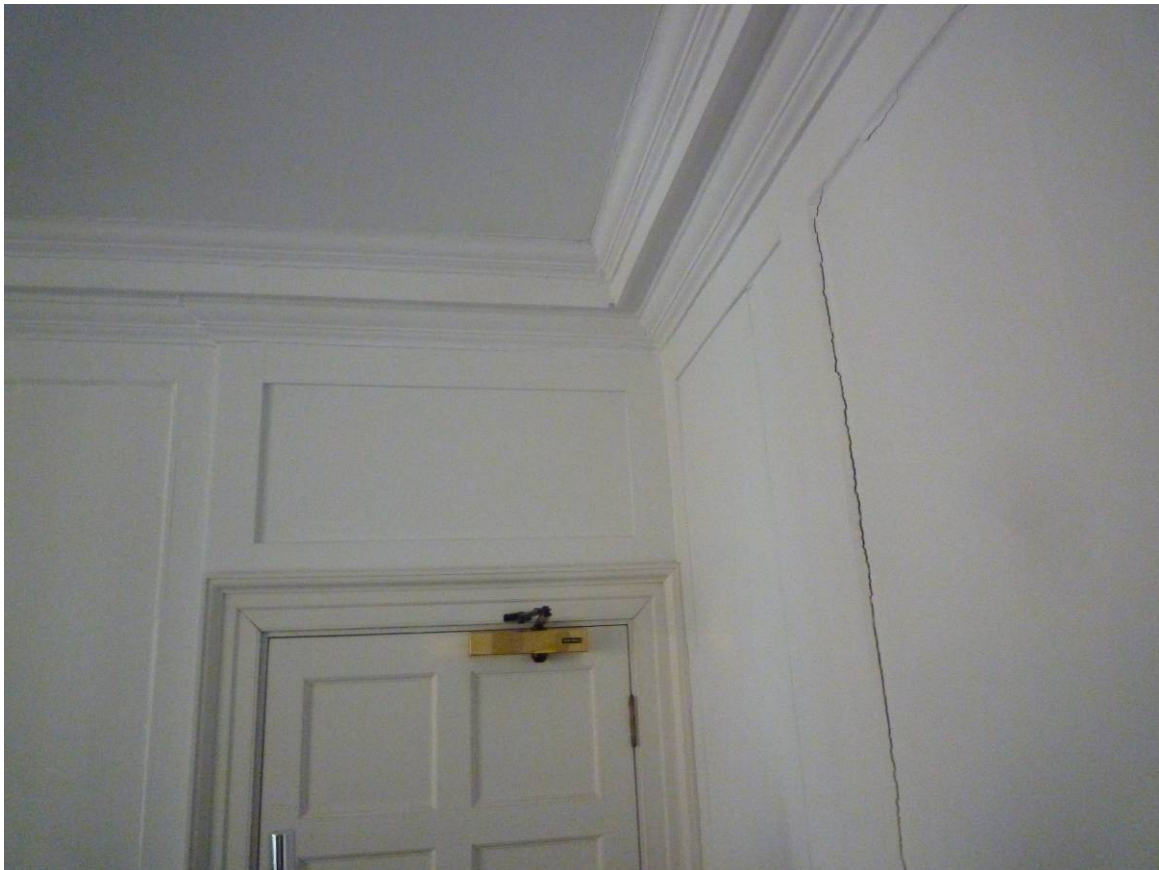
Fig. 36 Panelling in the second floor rear room
