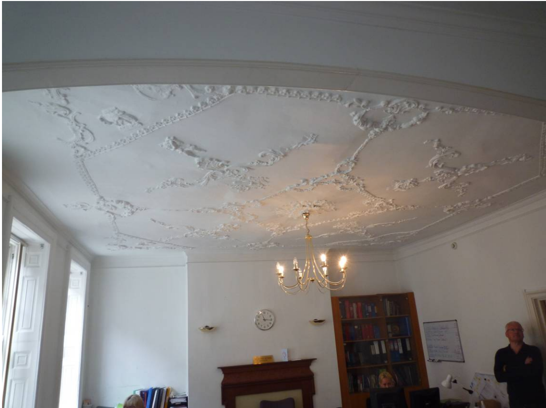
Fig. 37 Ceiling in first floor front room, from the south
