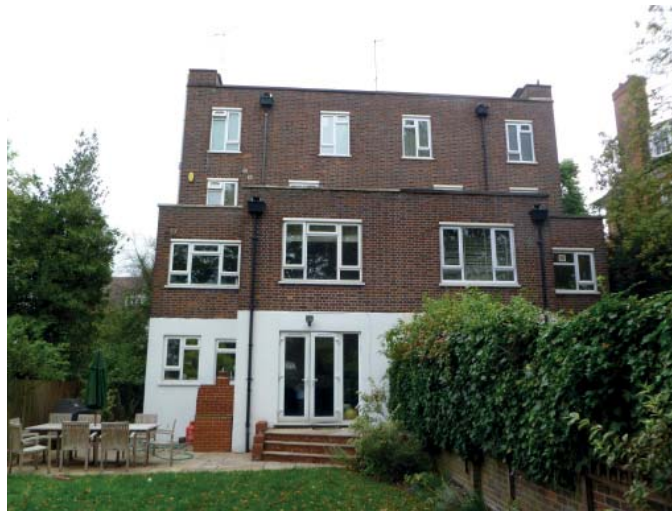
View from the rear showing no.19 obscured at garden level
