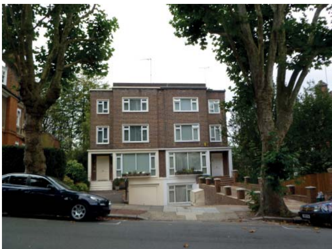
View from the street, no.21 is on the right
