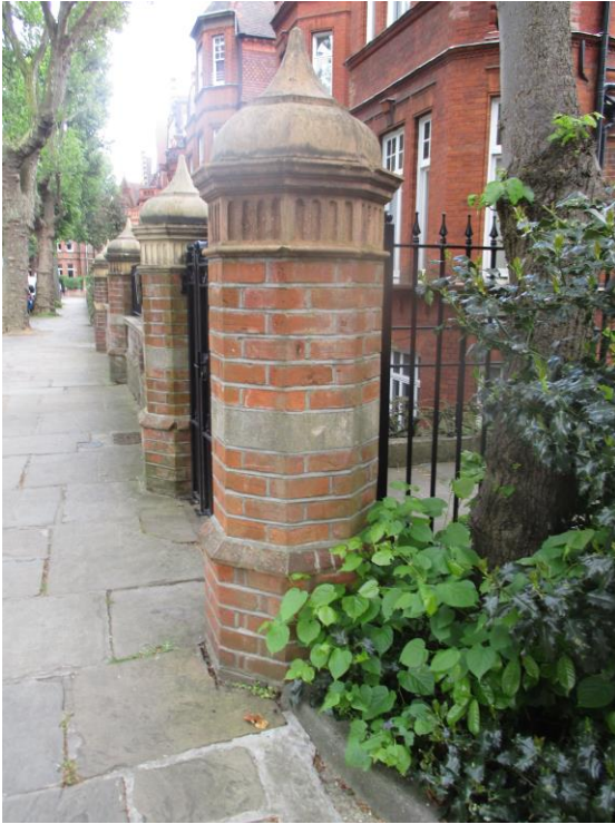
Photograph 3 – Existing left-hand pillar
