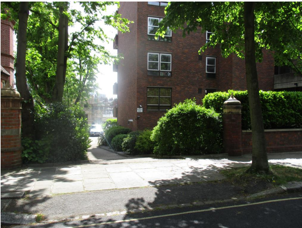
Photograph 2 – Existing vehicular entrance
