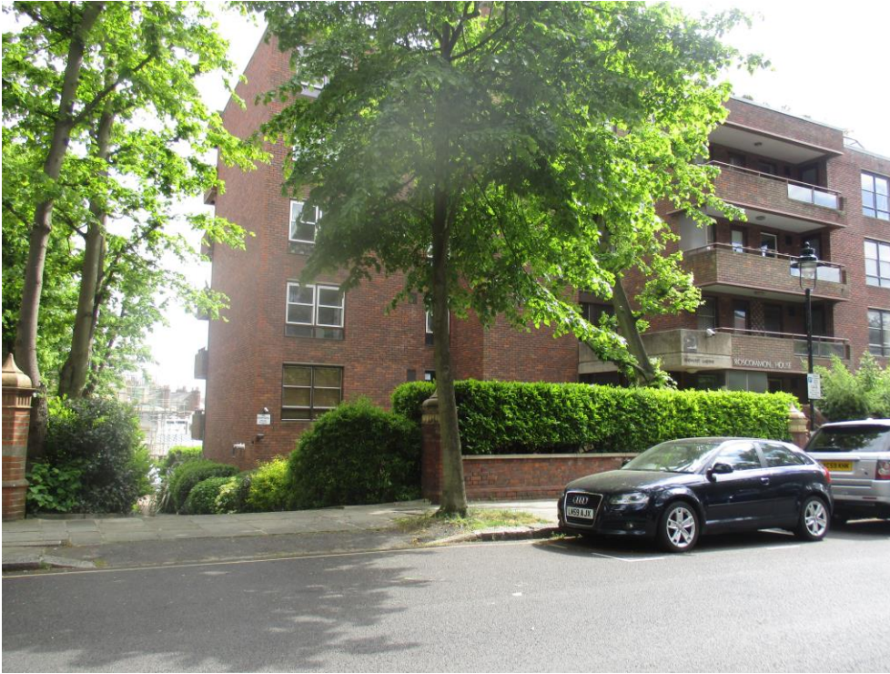
Photograph 1 – Front aspect of the property
