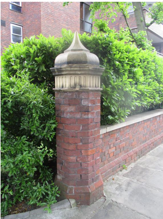
Photograph 4 – Existing right-hand pillar
