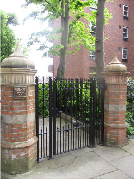
Photograph 5 – Existing gate No.4 Lyndhurst Gardens
