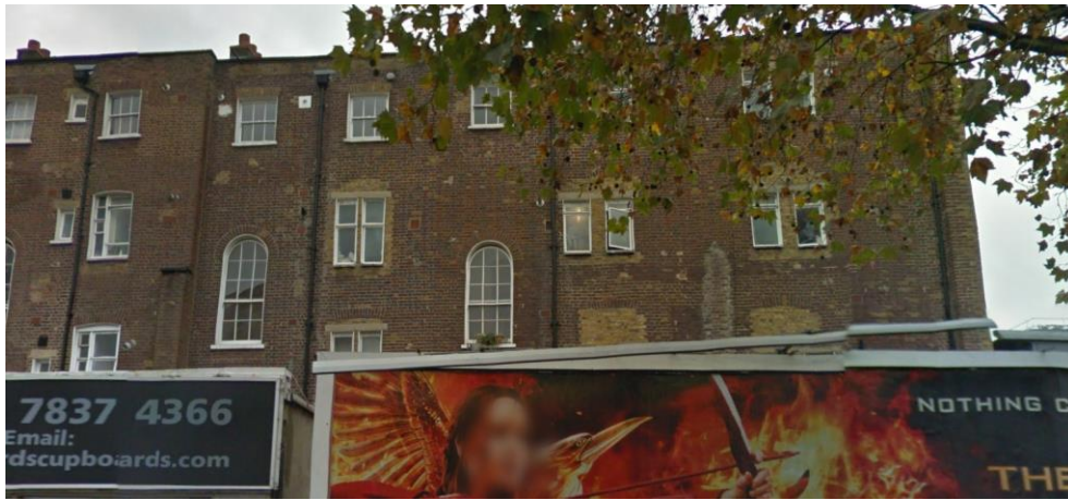
Rear View as seen from Gray's Inn Road
