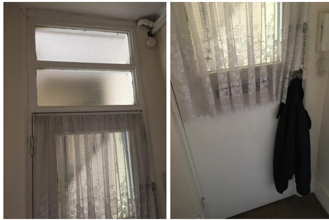
Photos: existing front entrance door to the flat
