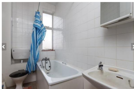
Photo of existing bathroom
