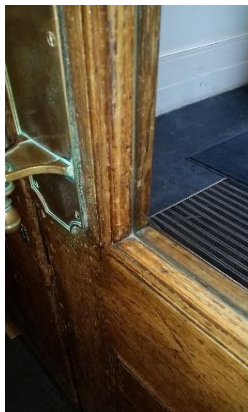
Existing multi pane 5mm float glass with flat section retaining beads and glazing bars
