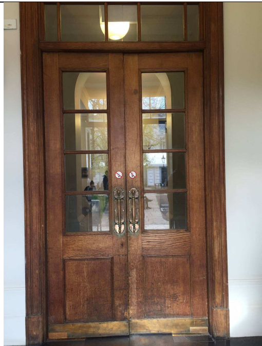
Photo 4: Typical condition of the door sets
