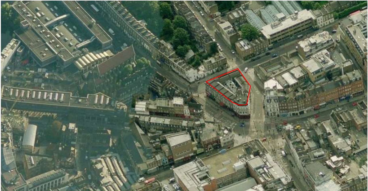
Figure 1- Aerial view of 174 Camden High Street
