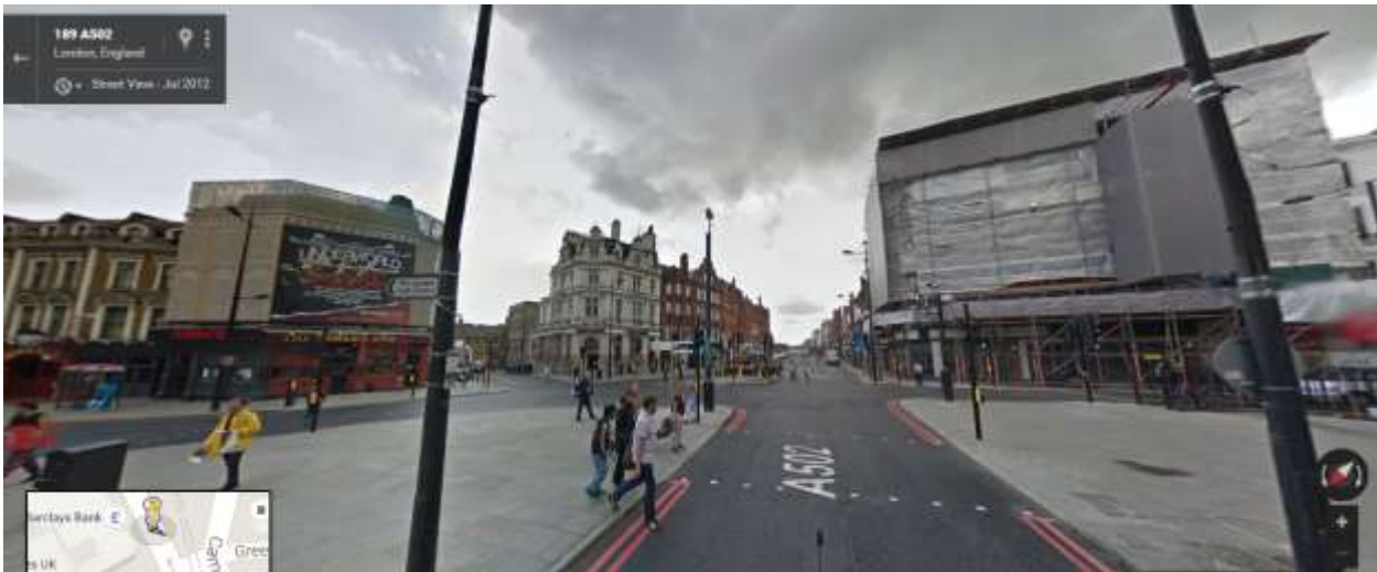
Figure 18 – Photograph from 2012, for comparison of the effect on the conservation area. Application site was undergoing repairs and had shroud scaffolding. At the same time, ordinary scaffolding on the building opposite is applied
