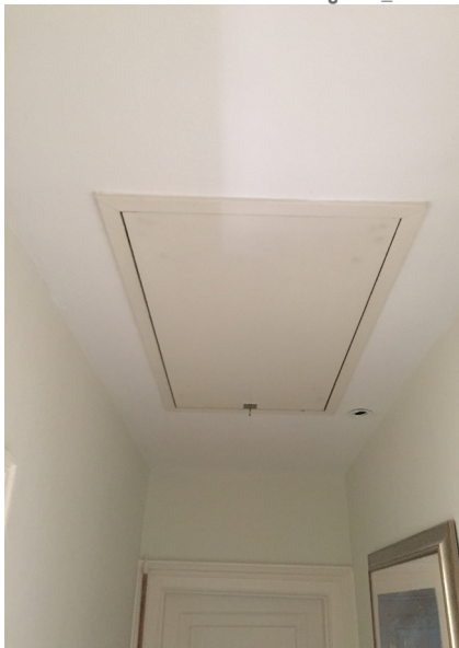
Fig. 12_ Corridor with ceiling hatch
