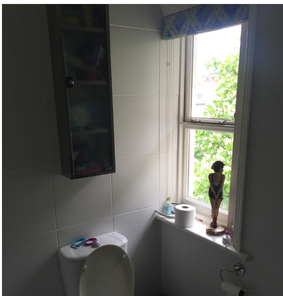
Fig. 8_ Split bathroom window
