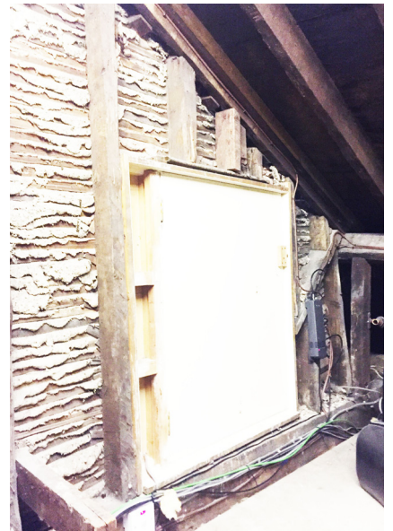
Fig. 14_ Loft hatch to balcony
