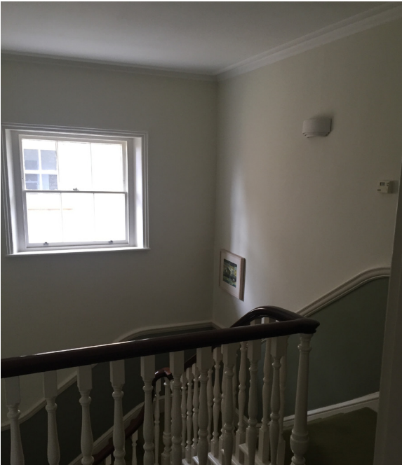
Fig. 10_ Stair well at top floor
