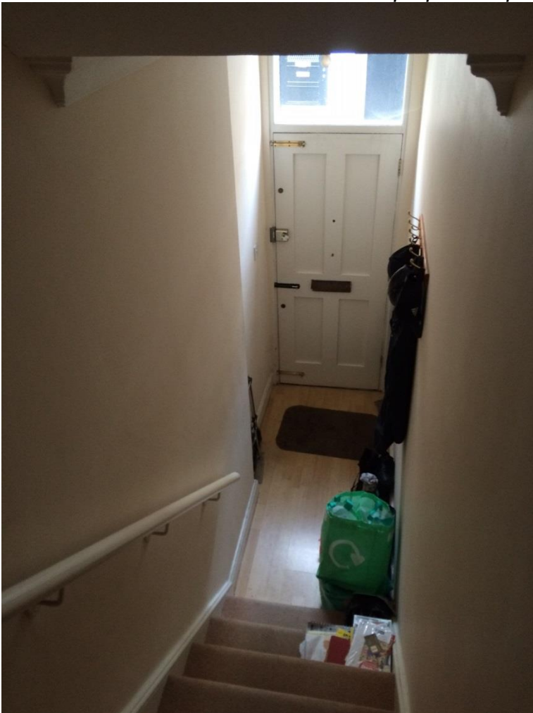
4. Entrance to first floor and location of proposed opening into ground floor
