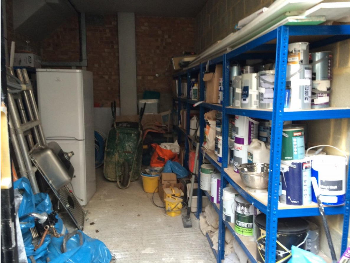
3. Ground floor internal (no.12)
