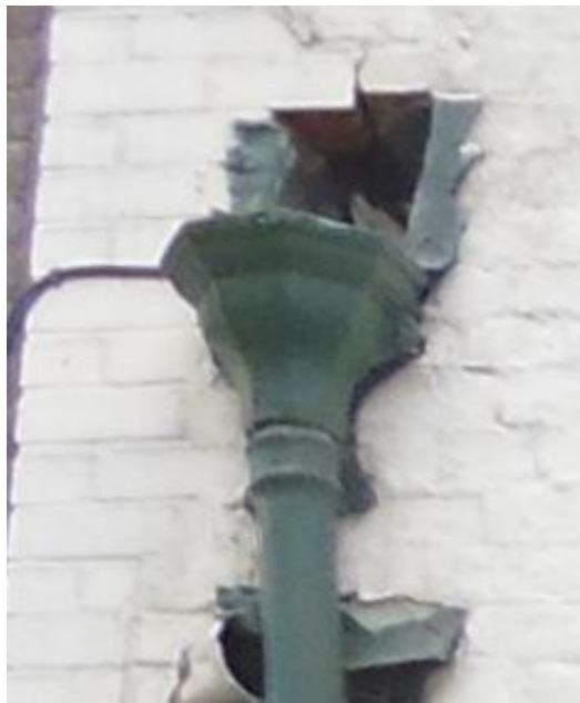
Fig.17 Detail of cast-iron hopper head
