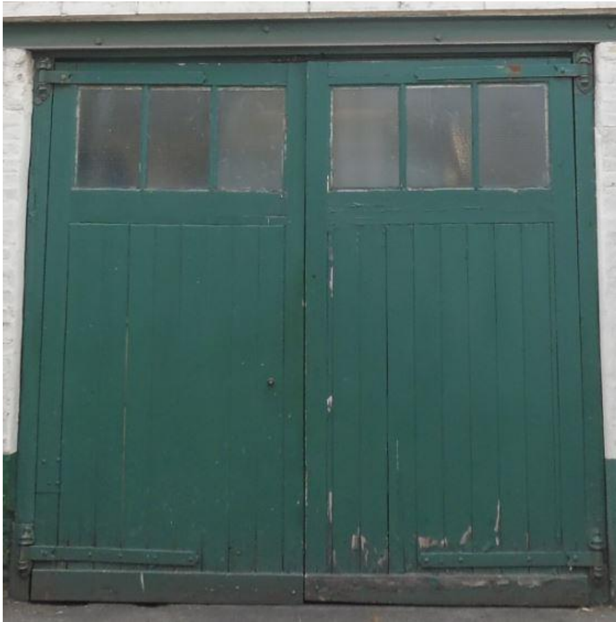
Fig.16 One of the double doors with Collinge hinges
