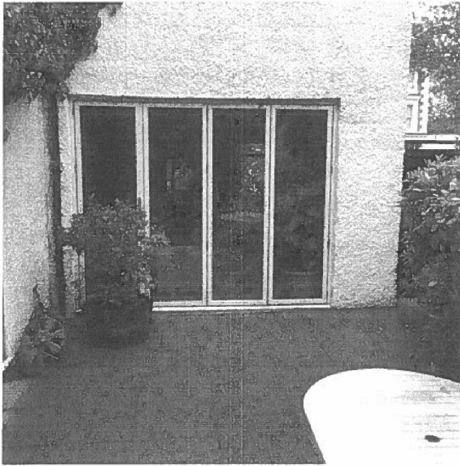
Rear patio windows to No. 76
