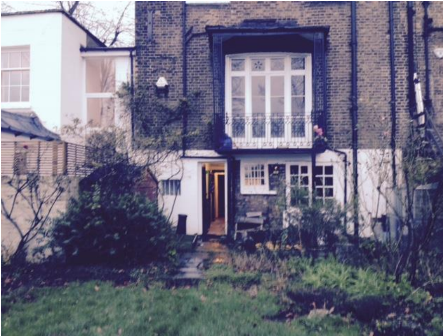
View of rear elevation
