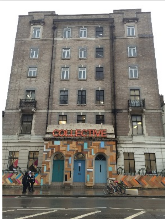
3. Insull Wing (Hampstead Road Elevation)
