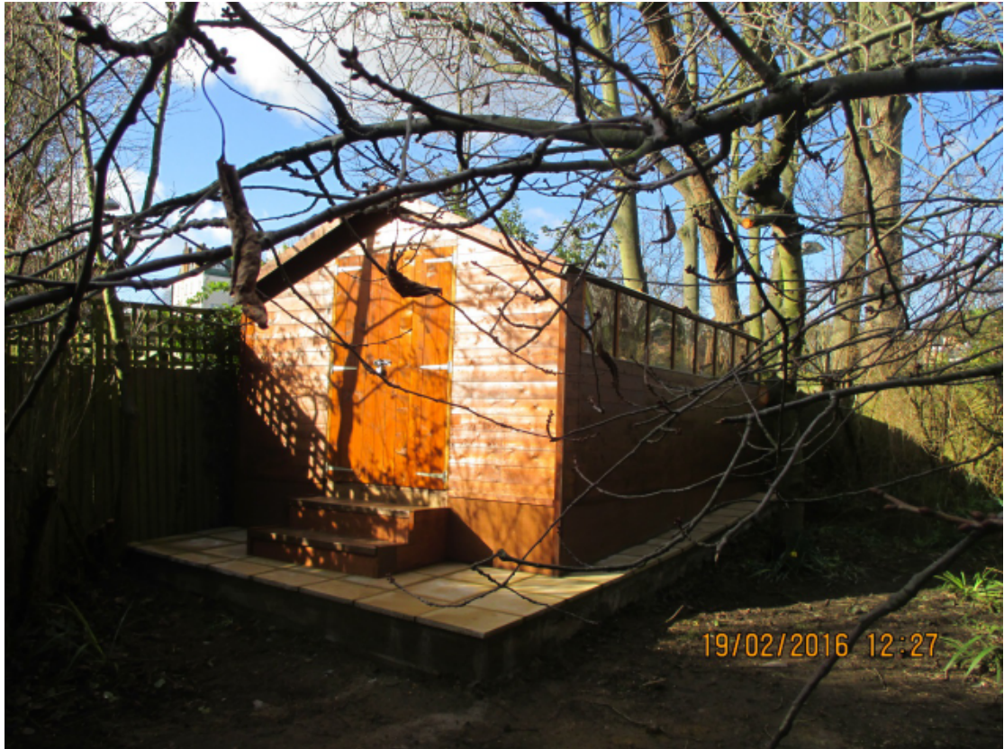
Photo 1- As built outbuilding
