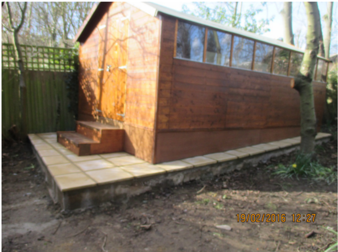
Photo 2- As built outbuilding
