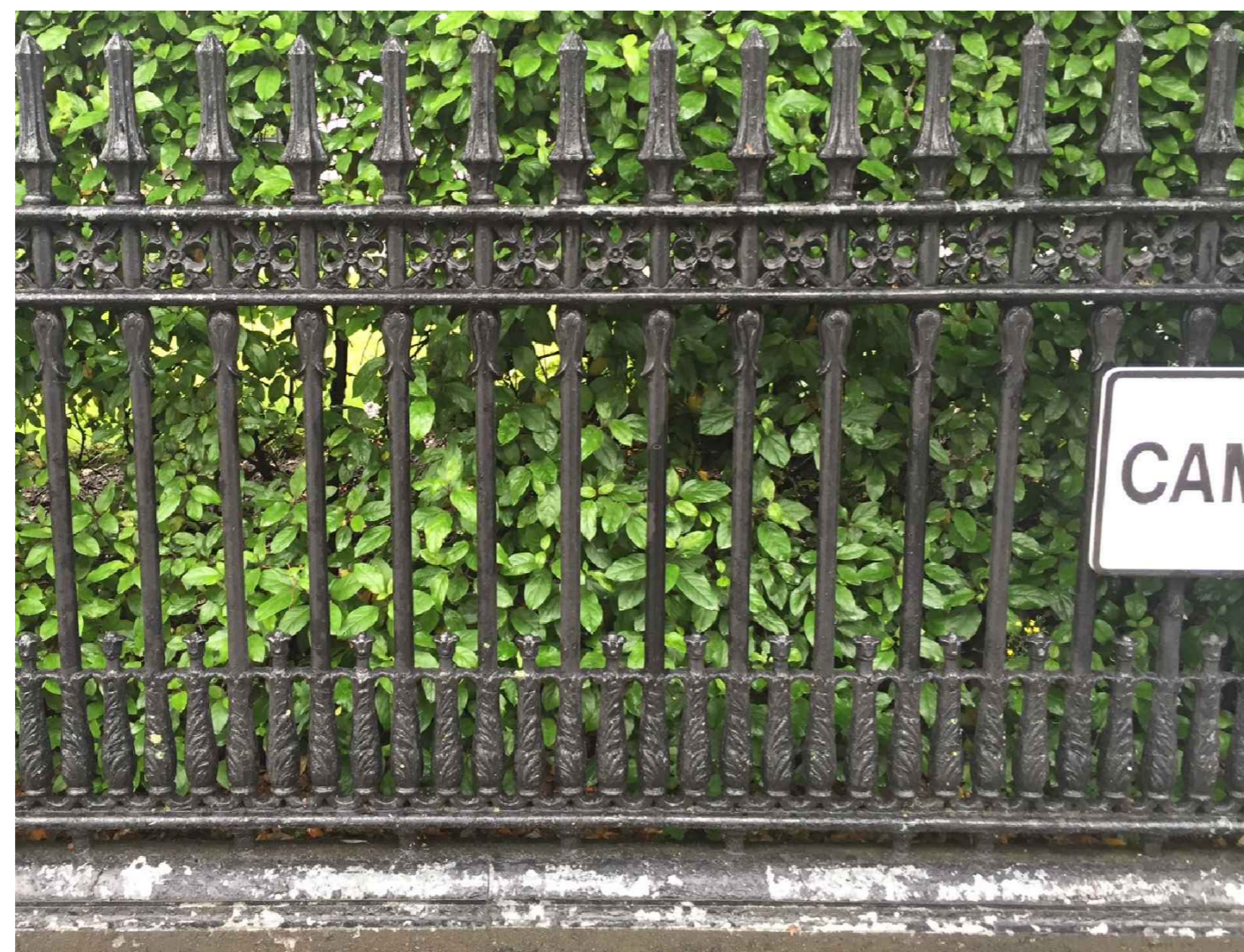
D-2 Photograph of existing RL.15 railings
