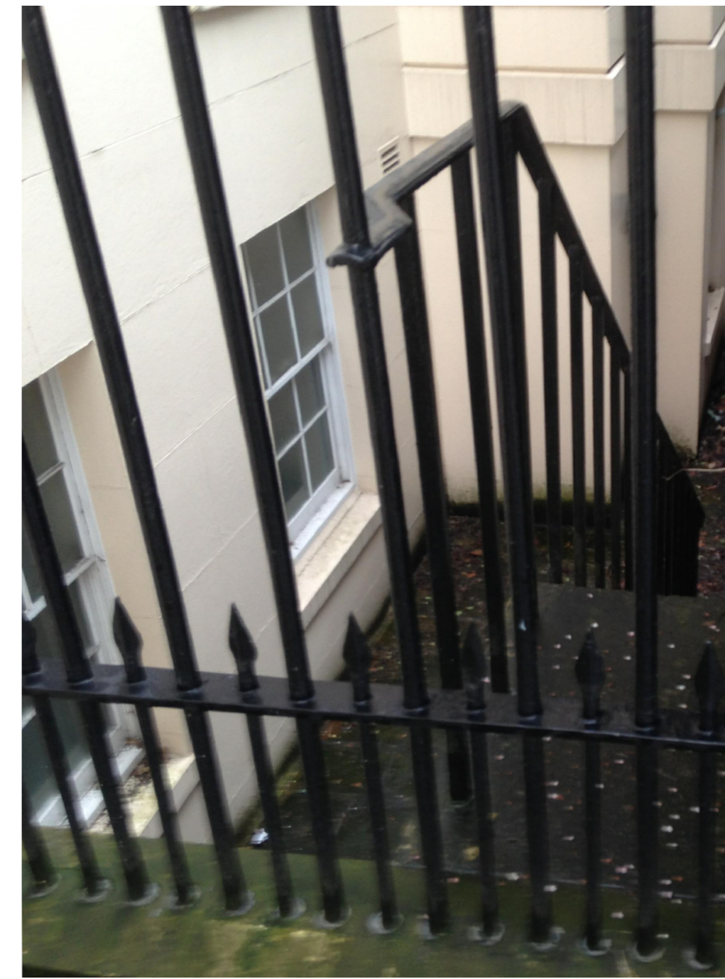
D-2 Photograph of existing RL.07 with dog rail detail
