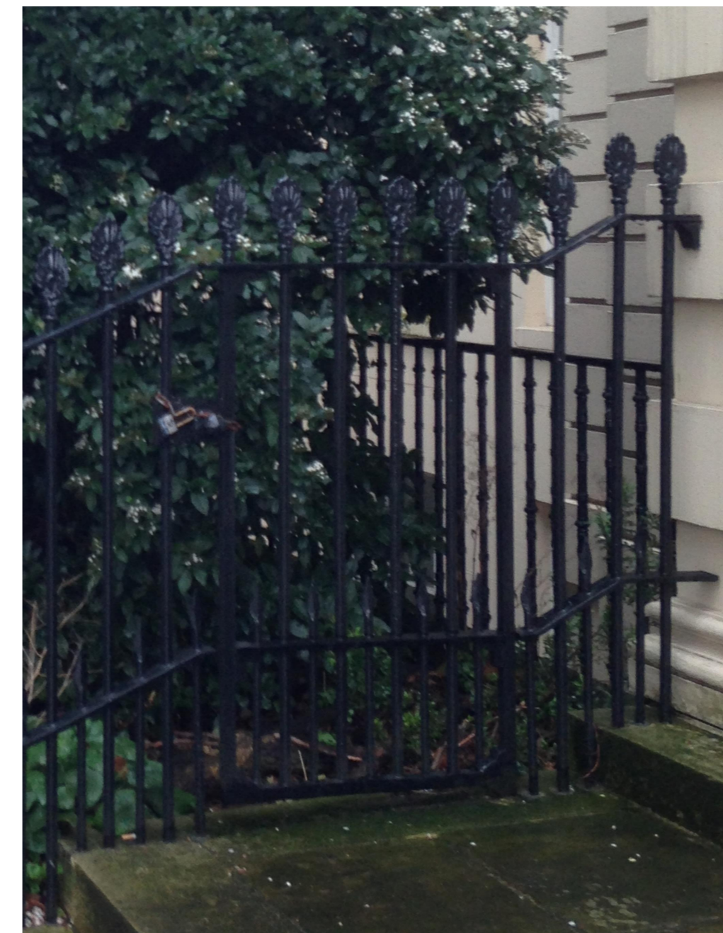
D-1 Photograph of existing RL.09 Railings with service gate
