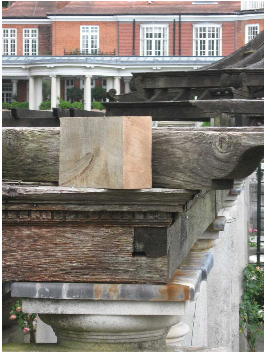
Photo of seasoned English Oak sample against 1990's oak beams and joists in the Pergola extension West of the footbridge
