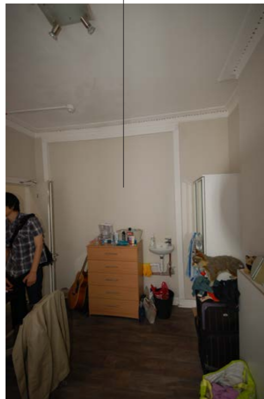
Ground Floor Bedroom: New Partition Wall Infil
