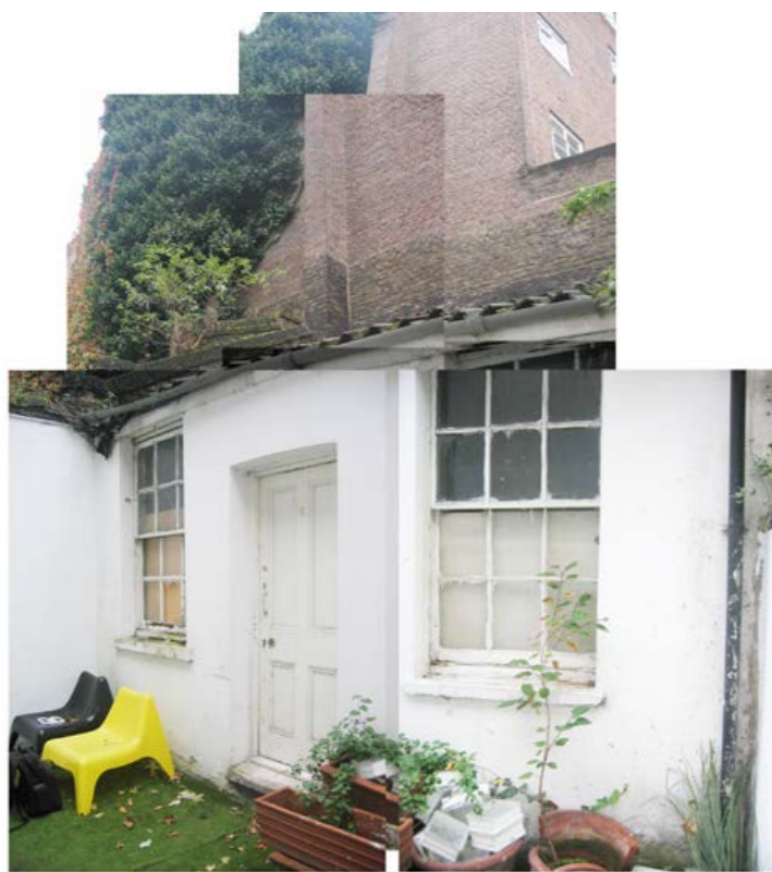
Existing Garden Annex
