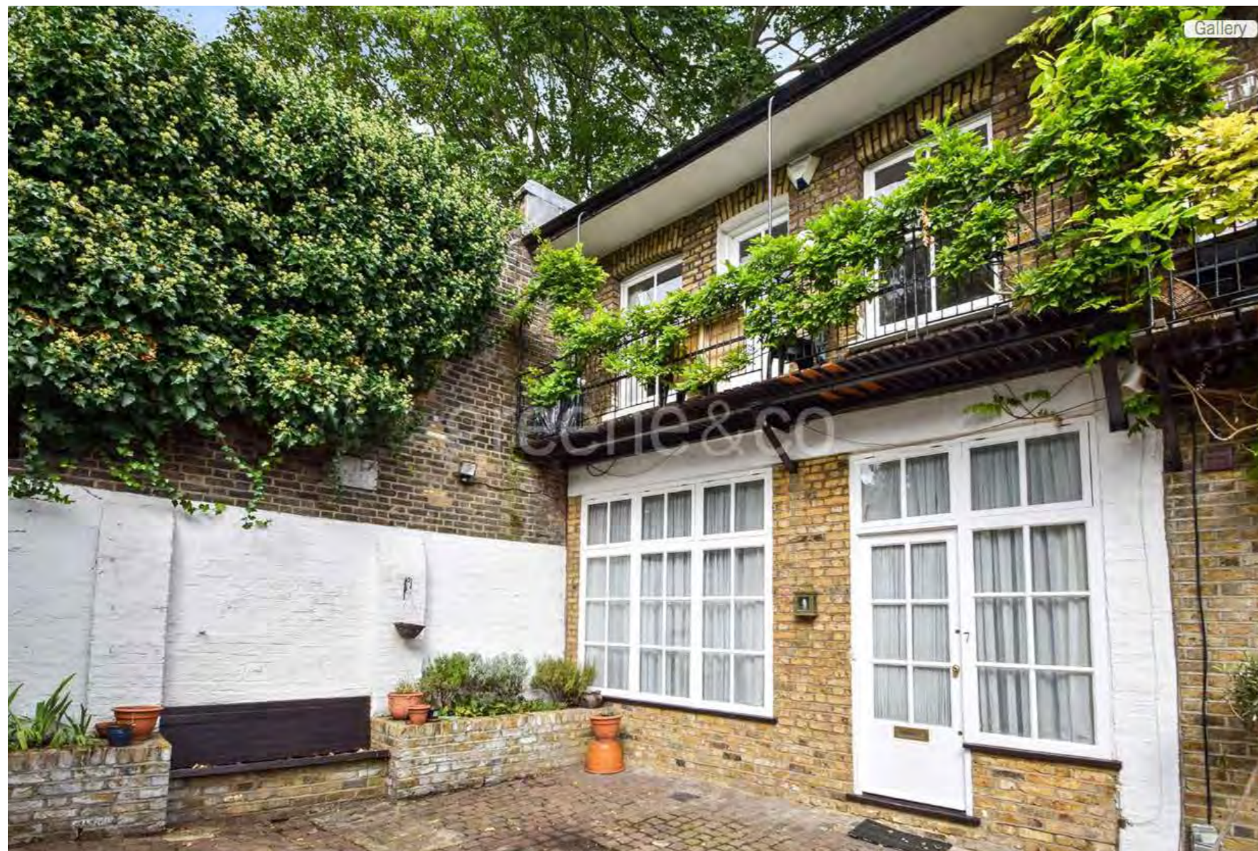
EXISTING FRONT FACADE
