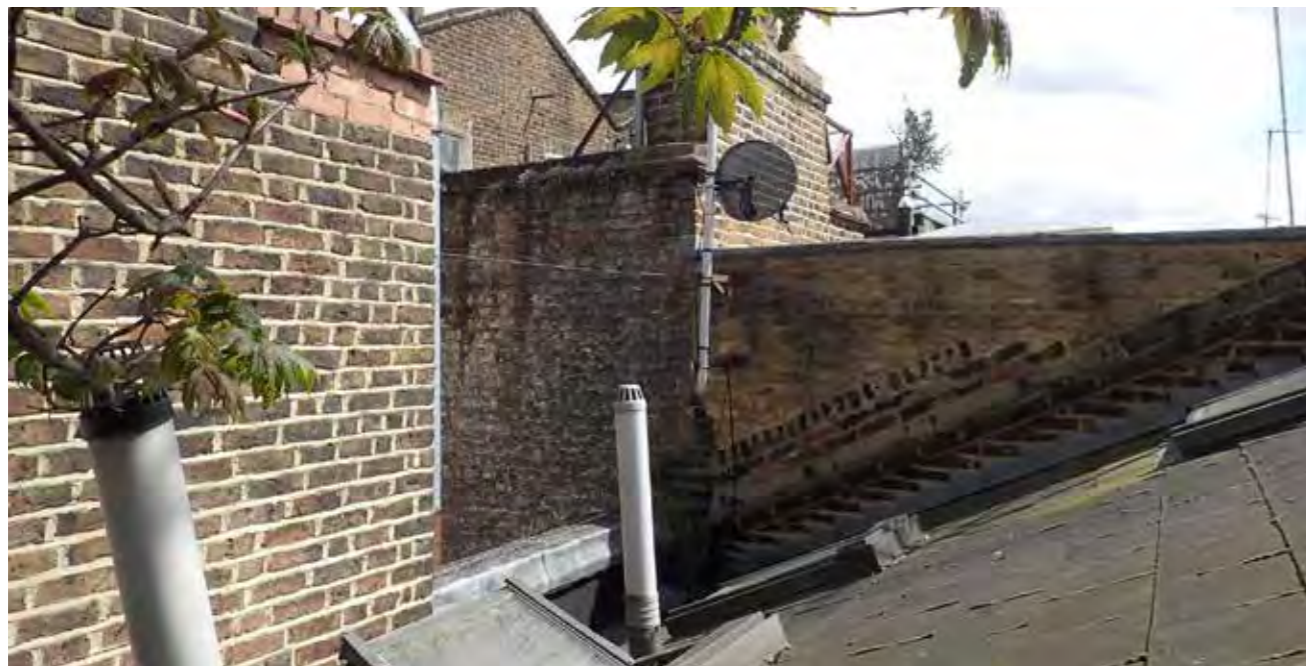
EXISTING ROOF SHOWING REAR NEIGHBOUR LIGHTWELL
