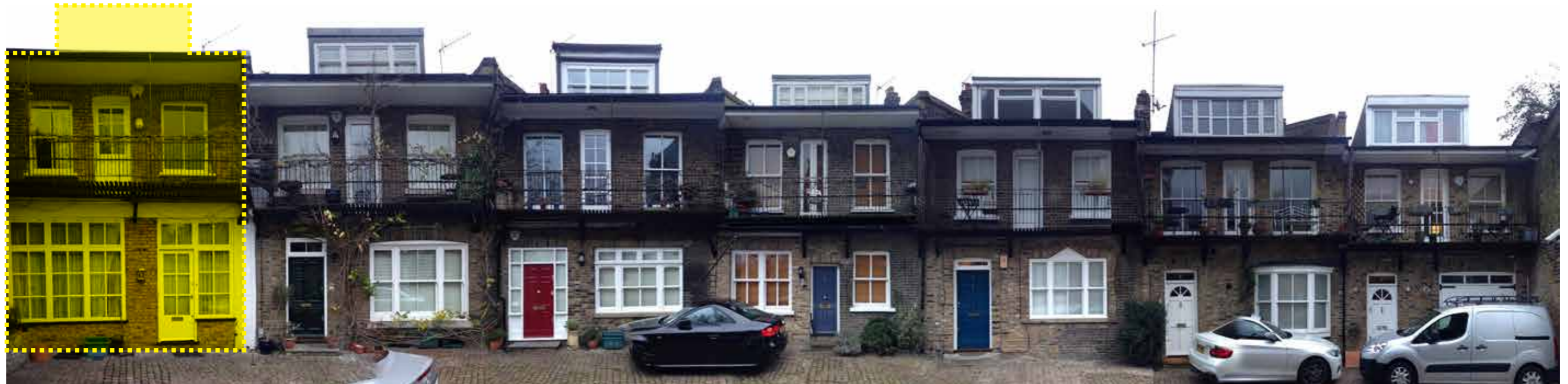
PHOTO MONTAGE OF STEELES MEWS 1-7 (RIGHT TO LEFT)
